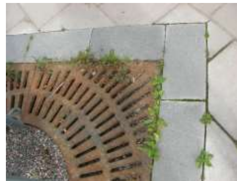
Natural materials used in collaboration with contemporary interventions creates a harmony firmly set in the past but with an exciting subtle twist. The uneven nature of the cobblestones sit against the steel edging and resin stone to form the tree surround.
