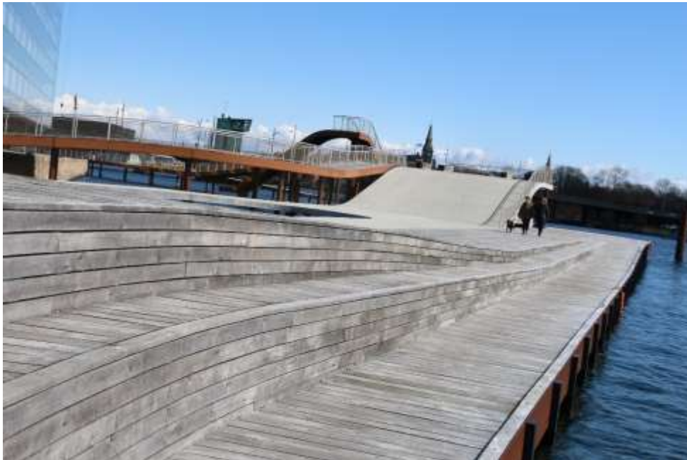
The clean sharp lines of the new boardwalk contrast against the soft contours and the natural timber plank deck. As in Kings Cross, the step heights promote sitting rather than walking
