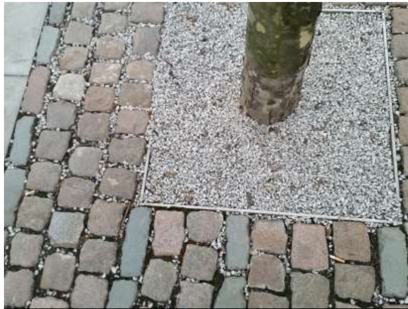
Natural materials used in collaboration with contemporary interventions creates a harmony firmly set in the past but with an exciting subtle twist. The uneven nature of the cobblestones sit against the steel edging and resin stone to form the tree surround.
