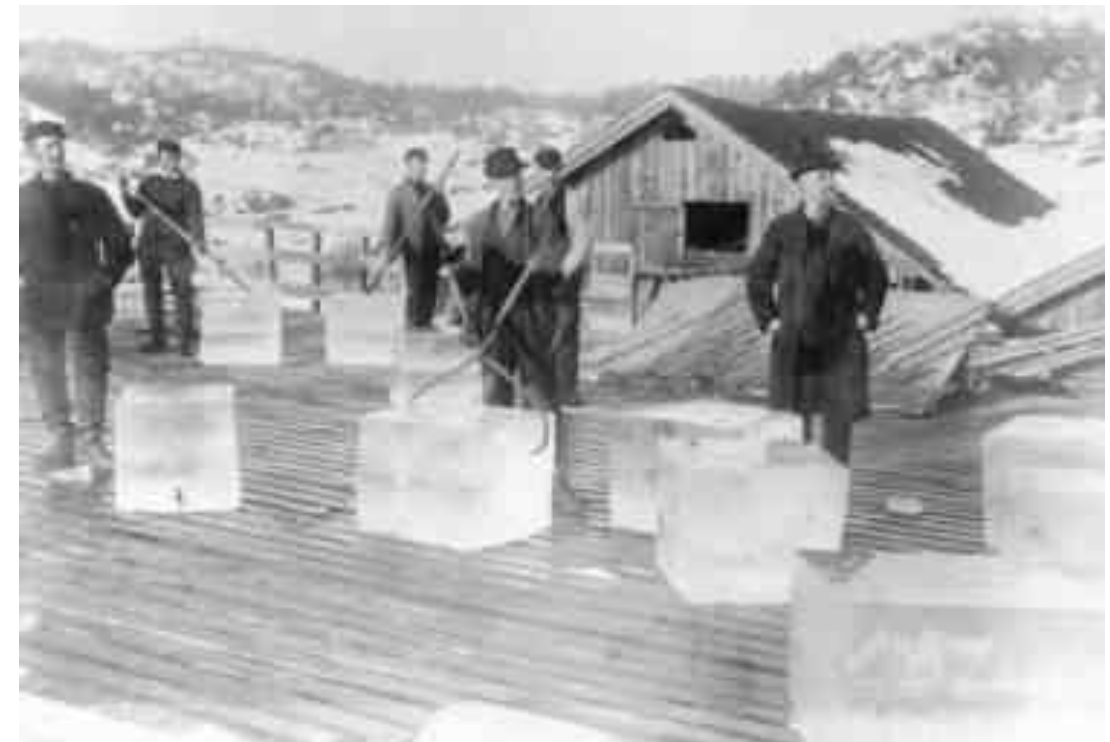
Ice cutting in Norway...Reference image for proposed sculpture; incorporating full scale human with ice blocks (Material to be agreed). Ice blocks to act as informal drinks shelves/tables
