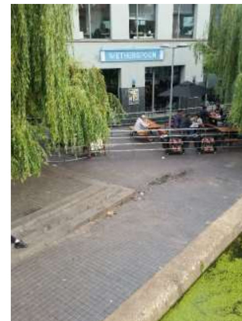
Site view from the bridge; the concrete kerb forms the junction between the ground and the canal
