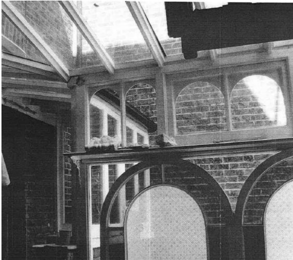
Rear extension across the full width of the 'well'.
