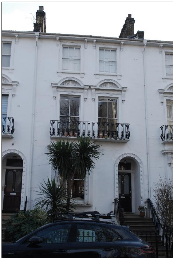
Front elevation showing windows & balconies.
