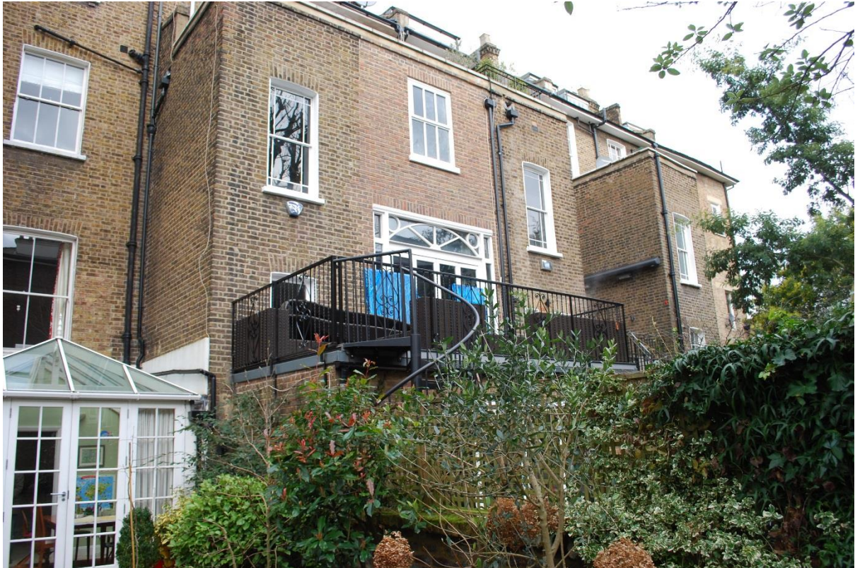
View of rear extensions to east.
