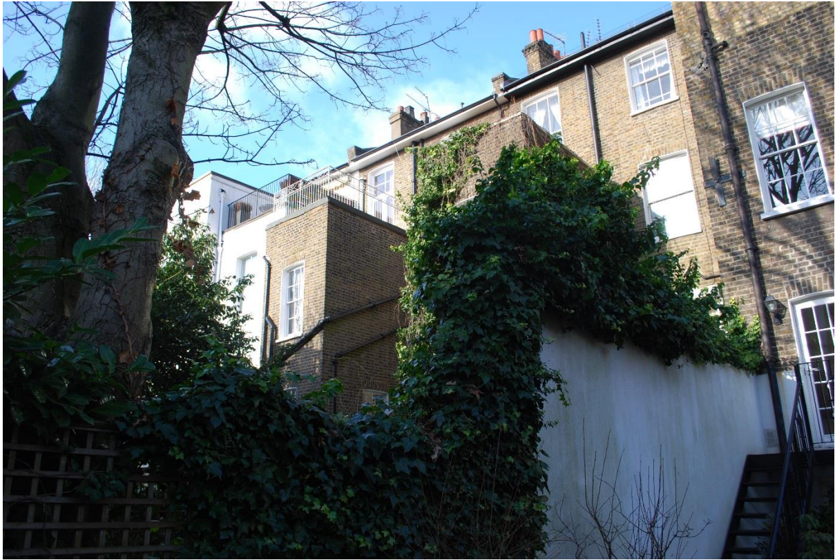
View of rear extensions to west.
