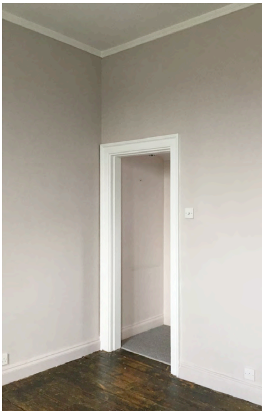
Ensuite Bathroom timber cornice and plaster ceiling
