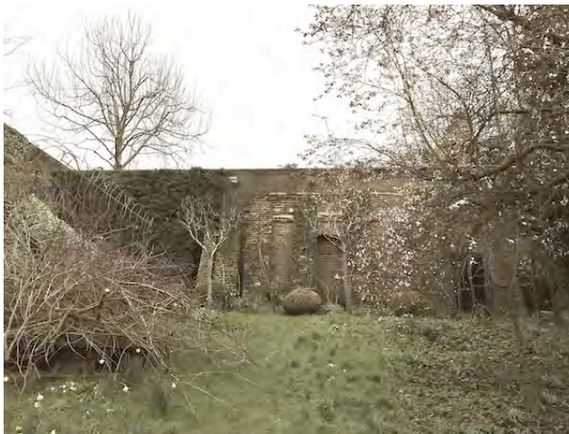
Rear retaining wall from lower garden/ west
