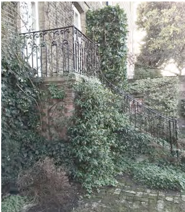
Stone staircase with wrought iron balustrade
