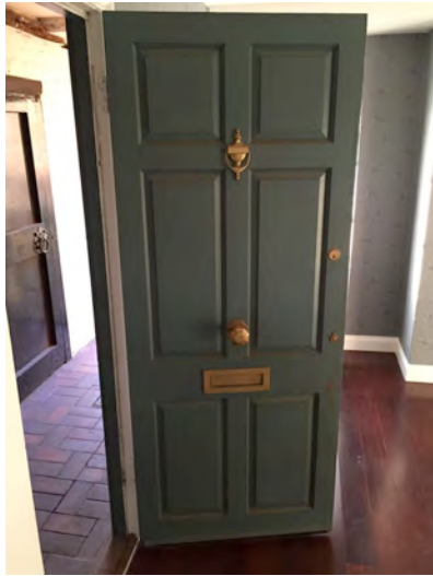
Extension/ Annex front door DLC1
