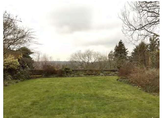
Rear retaining wall from upper lawn/ west
