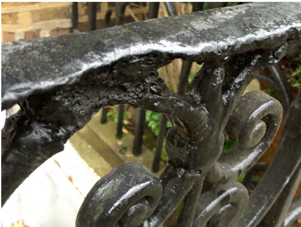
Front Ironwork detail
