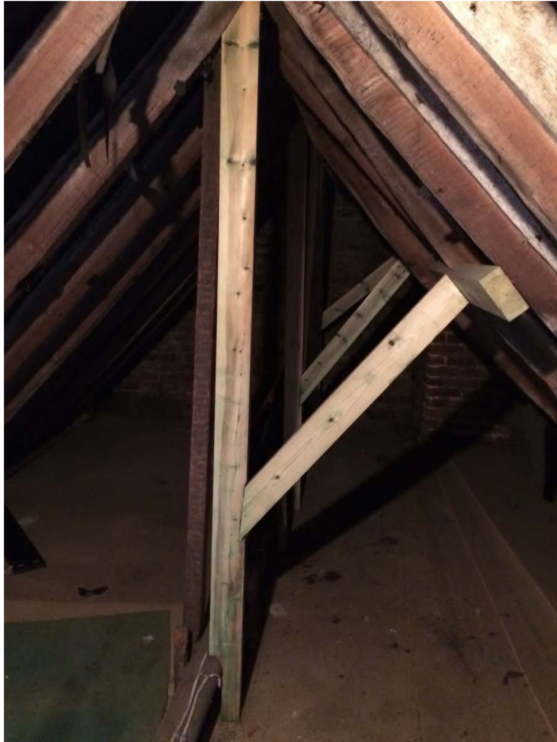
Photo 19 – Modern Repairs within roof space
