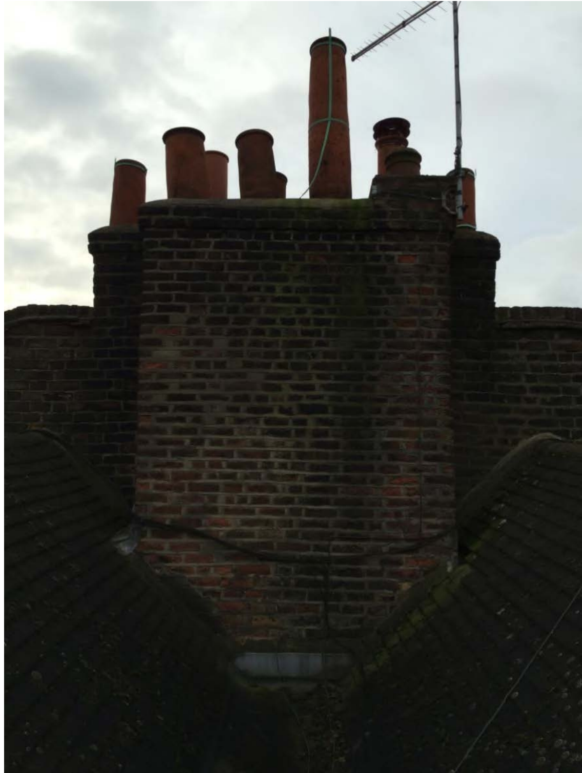
Photo 1 – Looking South to North elevation of southern chimney stack
