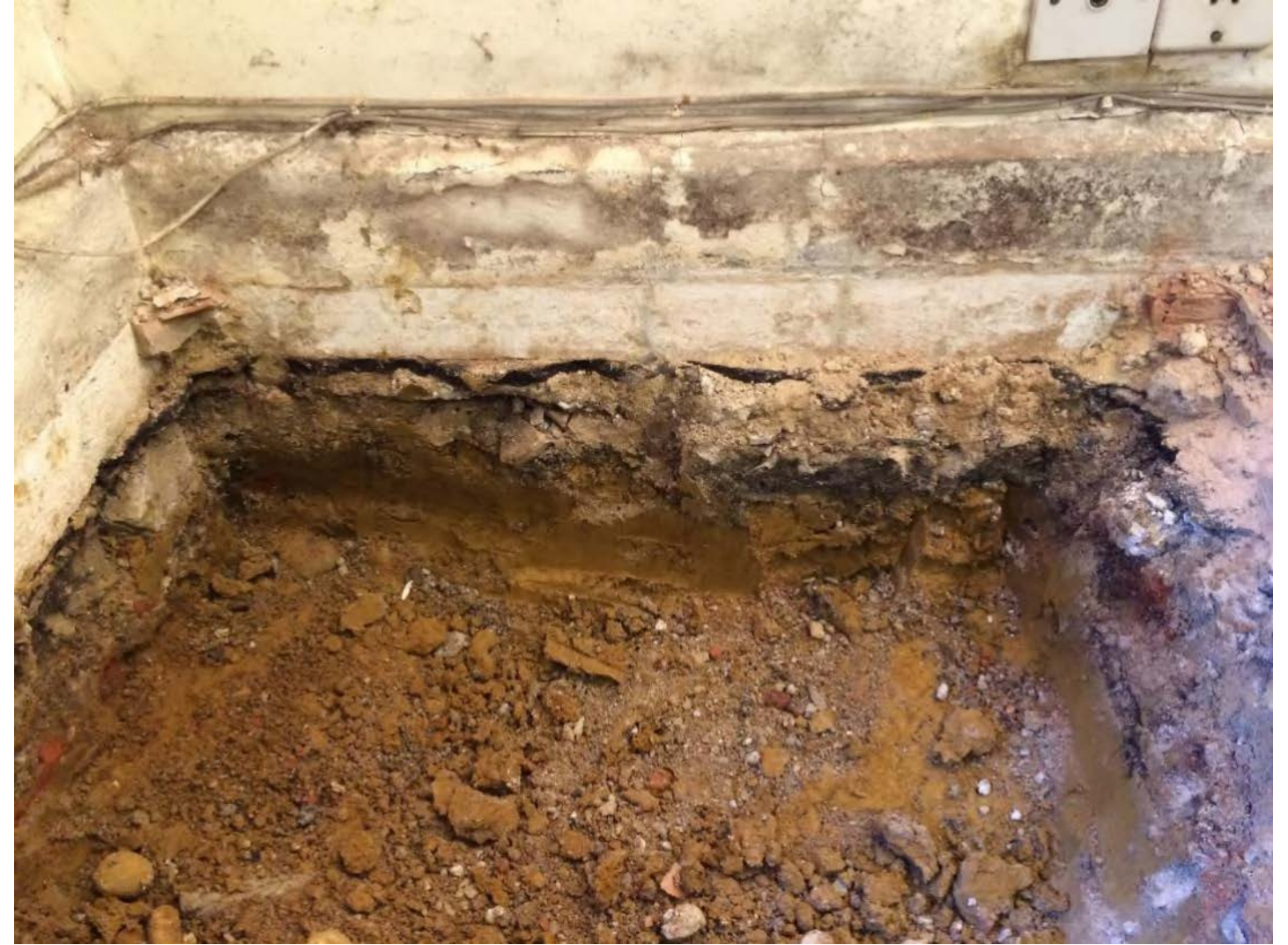
Photo 30 – Shallow foundations at lower ground floor level
