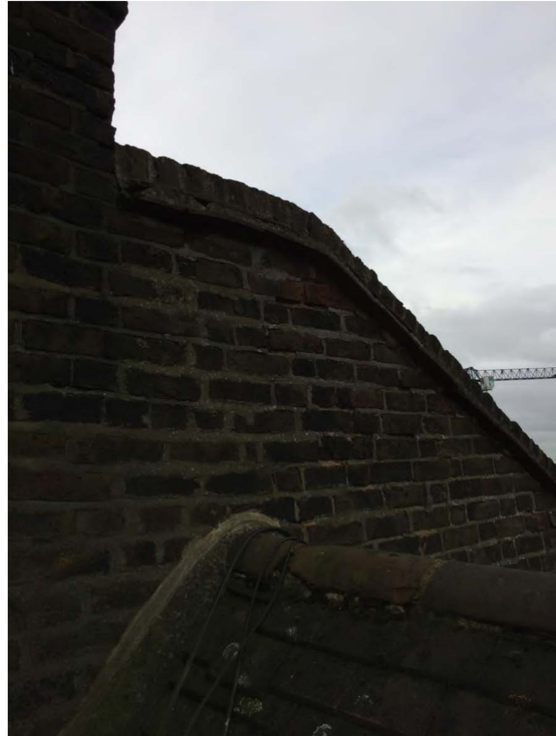
Photo 4 – Missing pointing on Party Wall parapet
