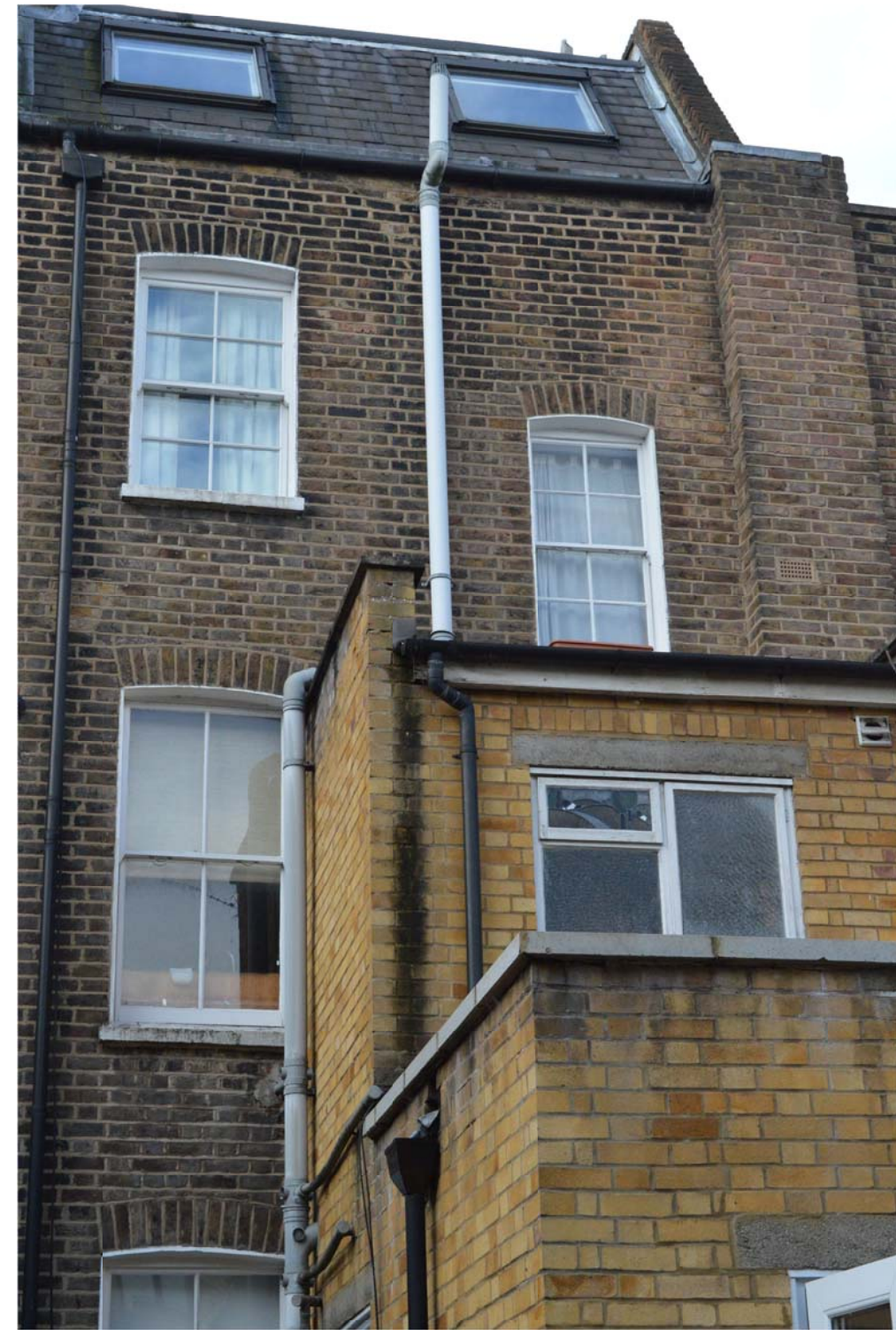
5 REAR ELEVATION - EXISTING PHOTO SCALE NTS
