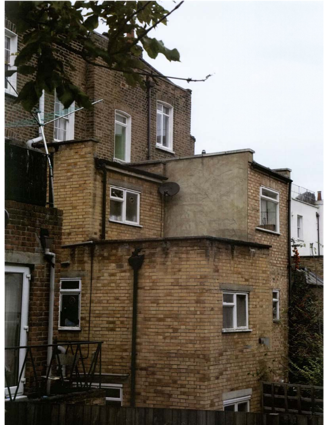
2 REAR ELEVATION - EXISTING PHOTO SCALE NTS
