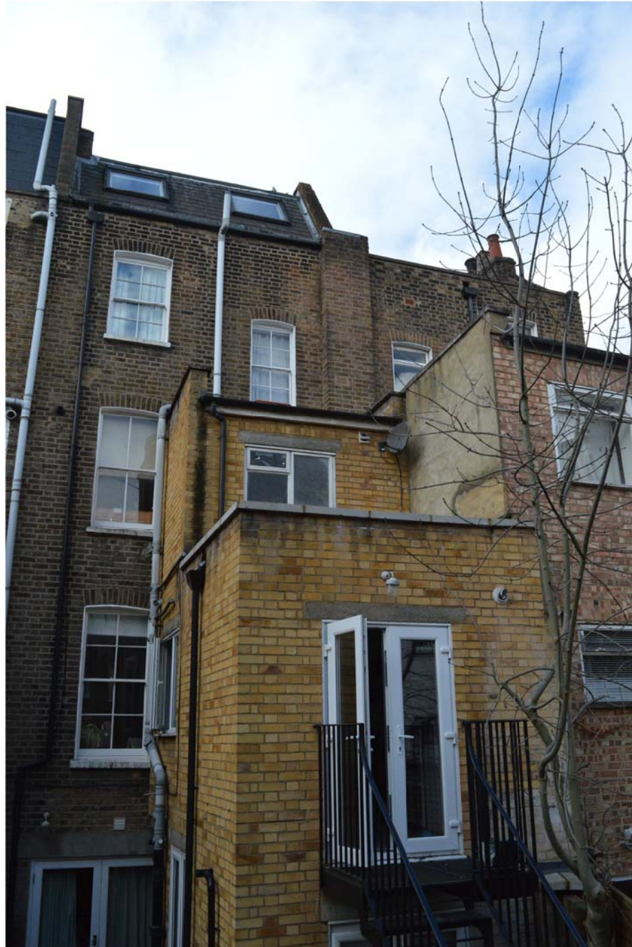
1 REAR ELEVATION - EXISTING PHOTO SCALE NTS
