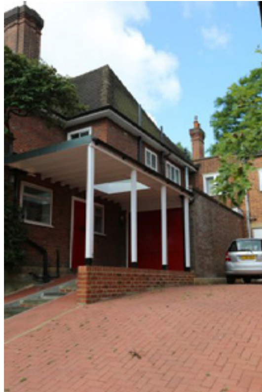
76 Lawn Road - only detached house in the grouping, four pane stair window, side car port, garage two storey garage wing behind
