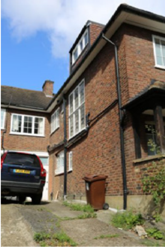
74 Lawn Road - six pane stair window, below eaves, dormer above two storey garage wing
