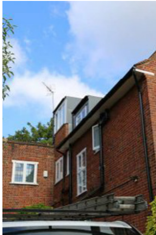
82 Lawn Road - four pane stair window, below eaves, two dormer bays above two storey garage wing
