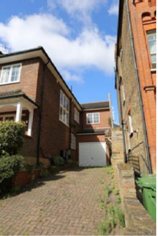
73 Lawn Road - six pane stair window, below eaves two storey garage wing
