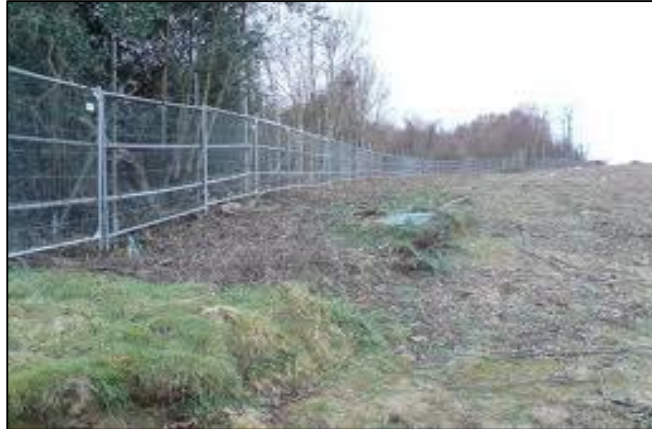
Tree protective fencing example
