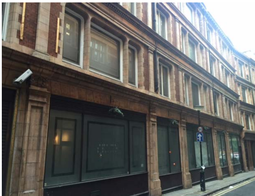
Front (west) elevation of 9-13 Grape Street
