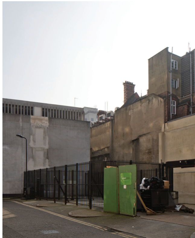
▲ Existing view looking South West from West Central Street
