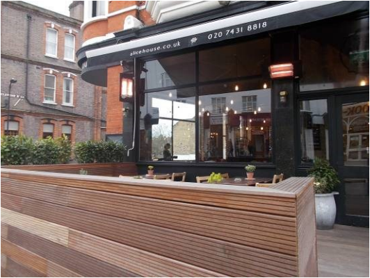
A view taken near the access point focusing on the detail of the of timber panelled enclosure
