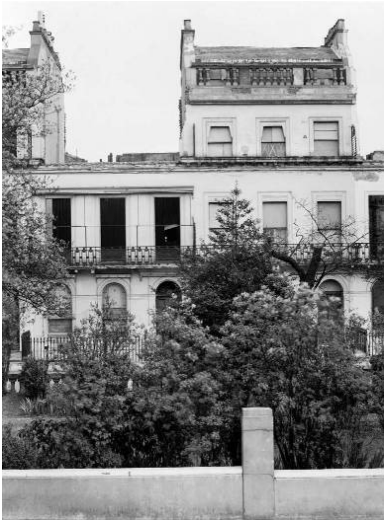
Figure 10. 35- 34 Chester Terrace, 1943 photographed by Herbert Felton. The terraces suffered collateral war damage and neglect.
