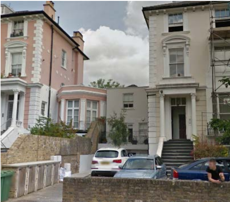
Fig. 4 Front Elevation of The Coach House No.102 Haverstock Hill. Image Copyright Google Streetview
