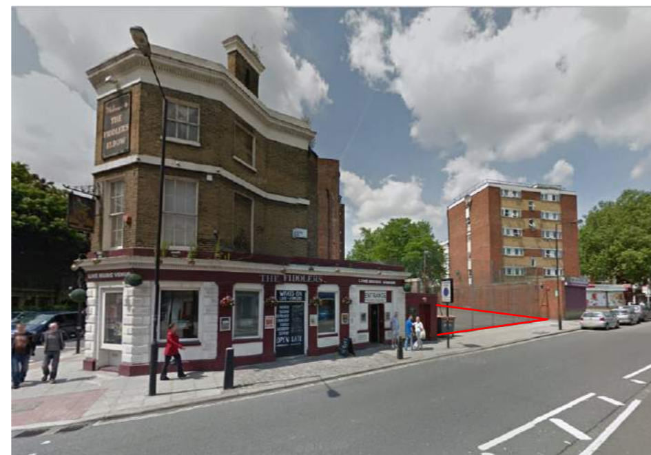
Figure 2: View ①, marked in Figure 1, looking northwest along Malden Road Site (left); the visible boundary of which is outlined in red.
