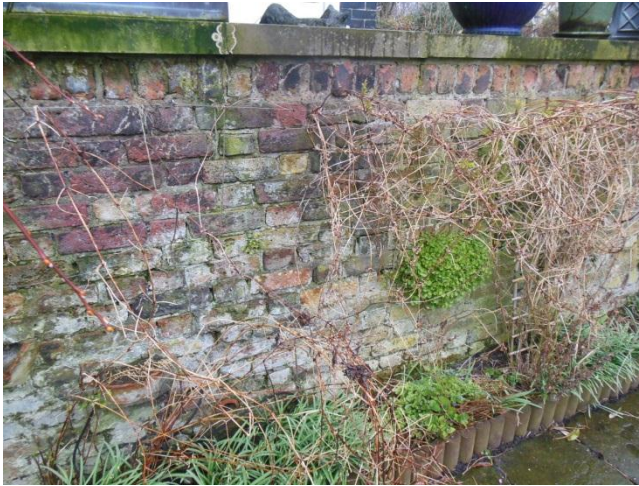
Figure 7: Poor condition of terrace retaining wall.
