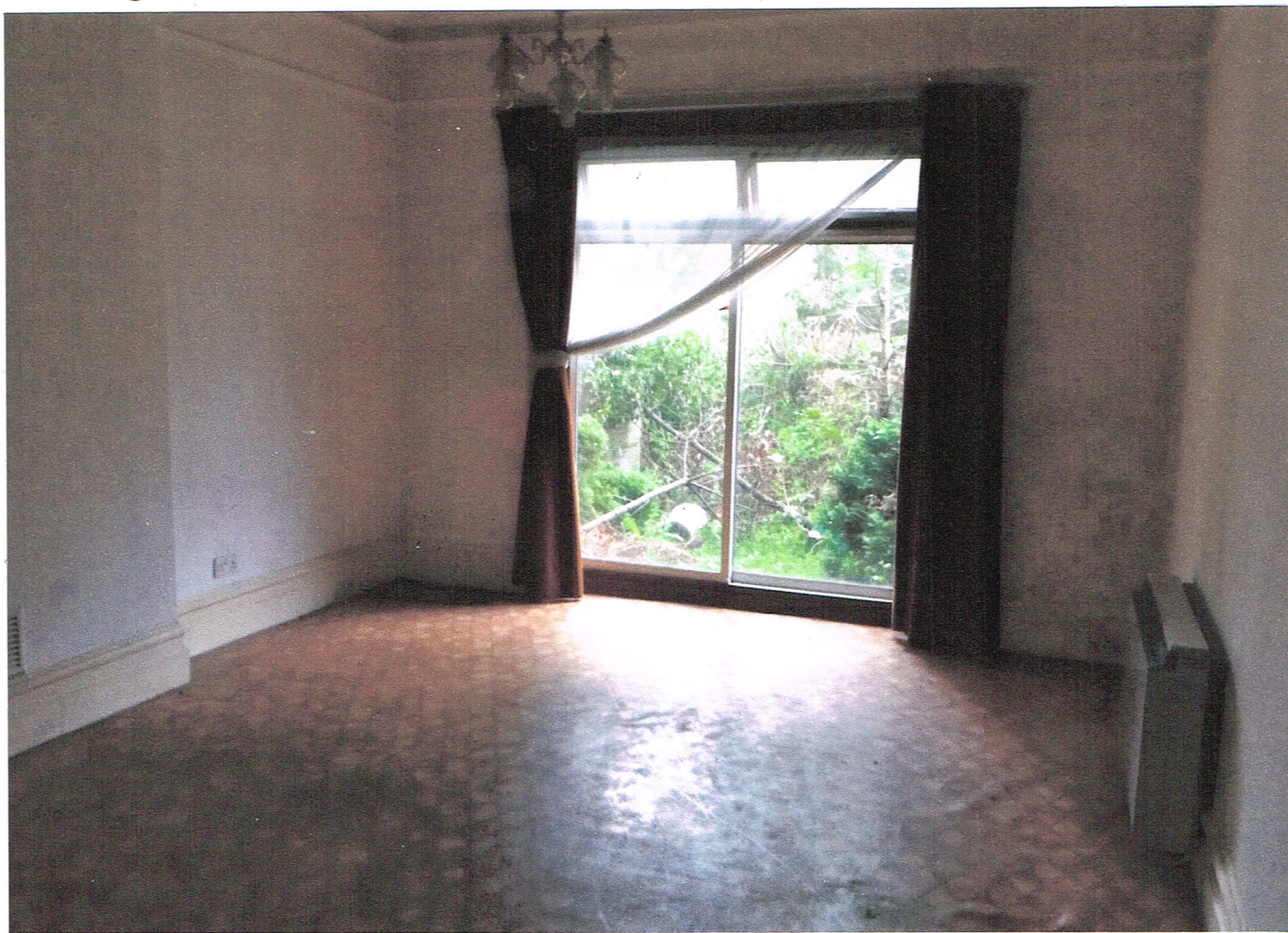
PHOTO 3 - Existing Metal Frame Sliding Patio Doors replaced
