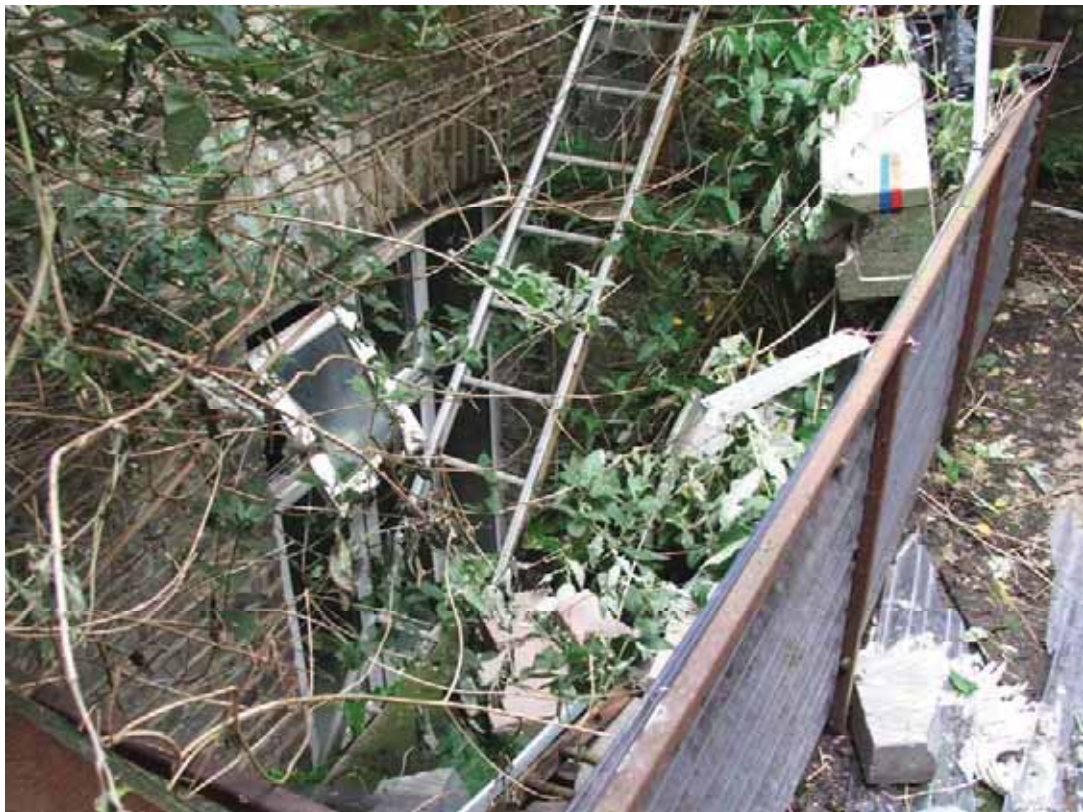
Figure 3.4: Lightwell to basement area (in yard)
