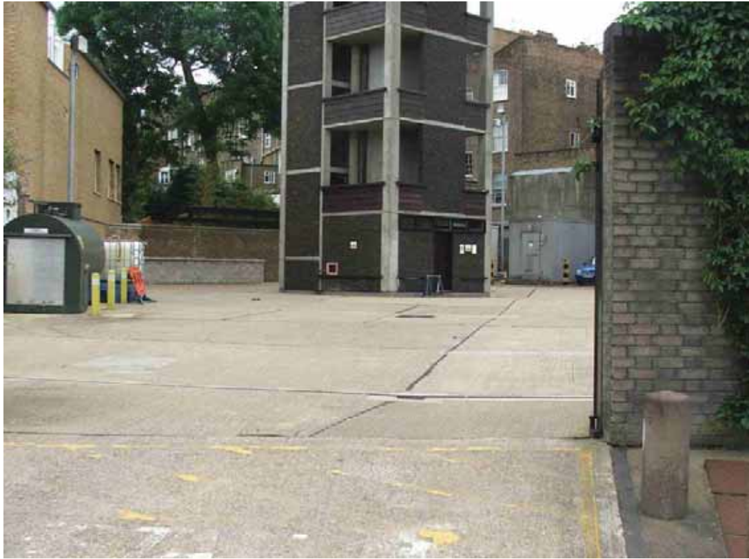
Figure 3.7: Off-site Fire Station, with fuel tank (LHS), practice tower (C) and generator (RHS)
