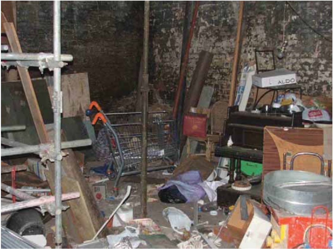
Figure 3.5: Internal view of outbuilding
