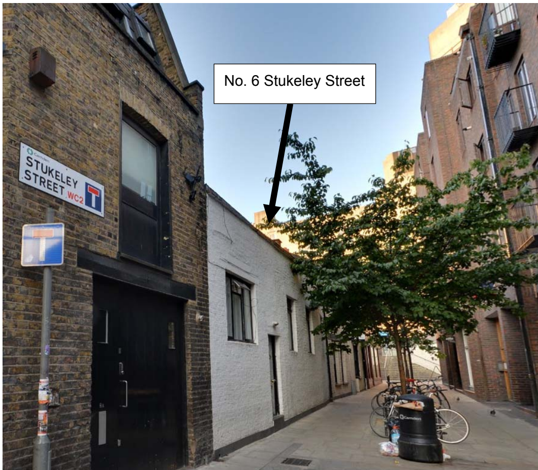
Figure 1 Street View Image of the site - July 2015
