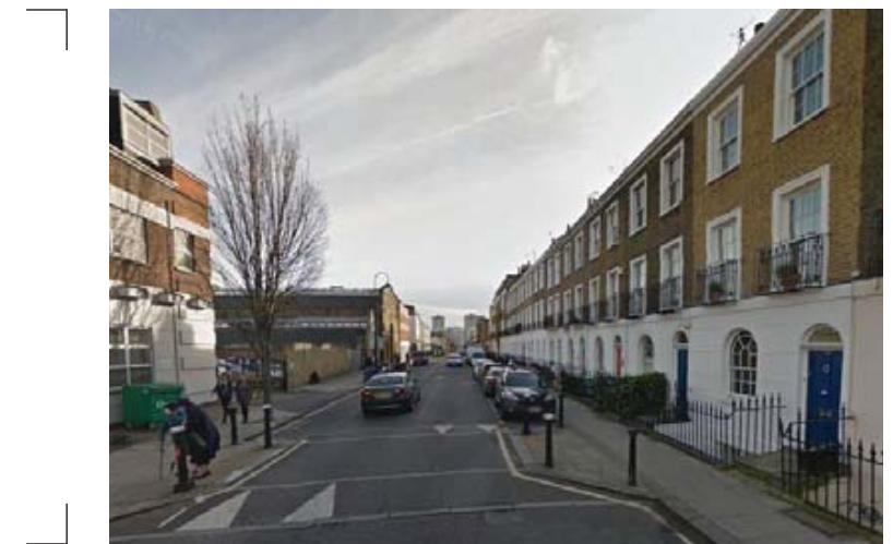
South View, 129 Arlington Road
