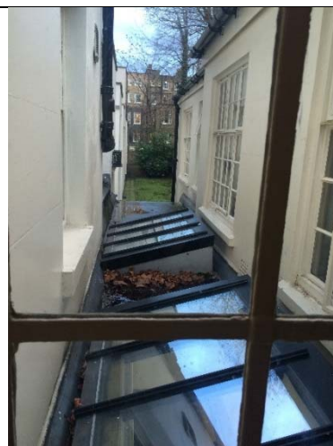
Fig. 04 - Existing Crittall windows to be replaced, overlooking an internal flat roof area.
