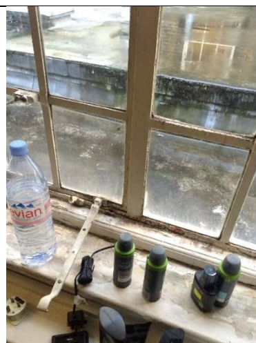
Fig. 06 - Existing condition of the Crittall windows to be replaced, overlooking an internal flat roof area.
