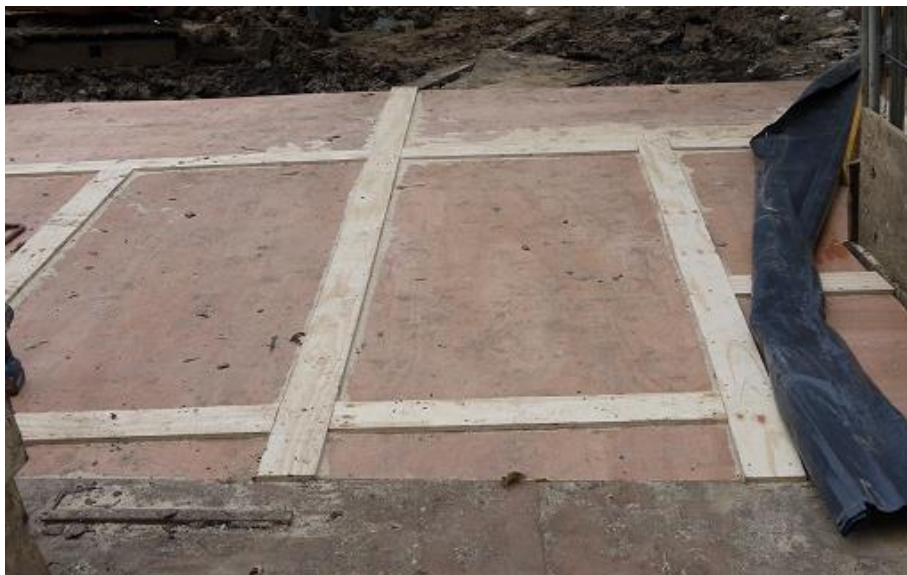
Figure 7. Plywood sheeting used as ground protection.
