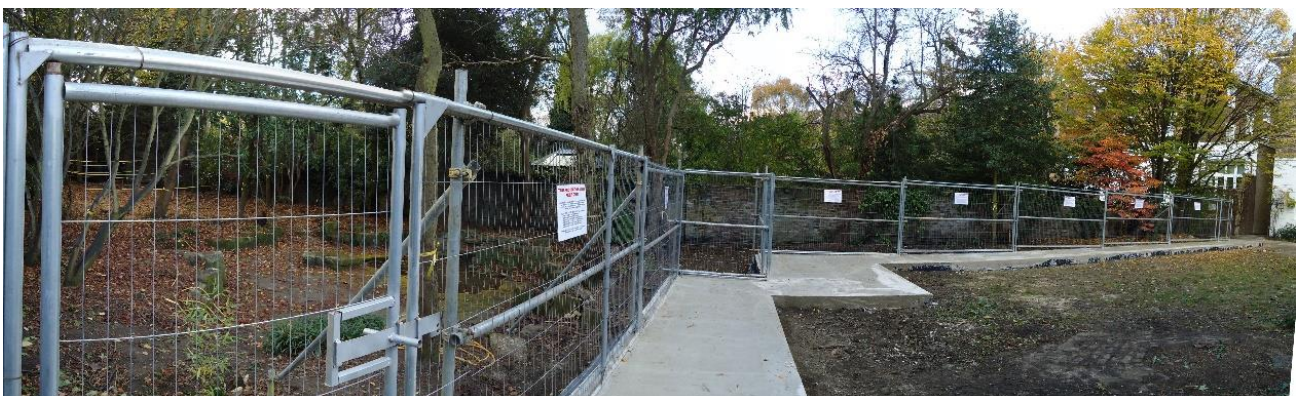
Figure 4. Photograph to illustrate installed protective fencing
