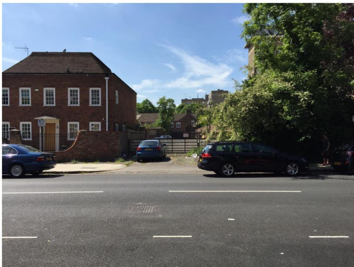
2. View towards the front of the site (with 1 St John's Wood Park on the left)
