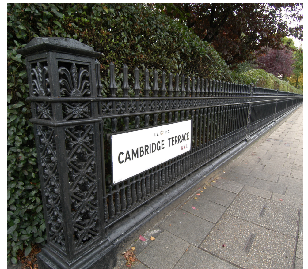
Photo no. 14 Box standard Listed Railings RL15 (part of EH list entry no. 1244298)
