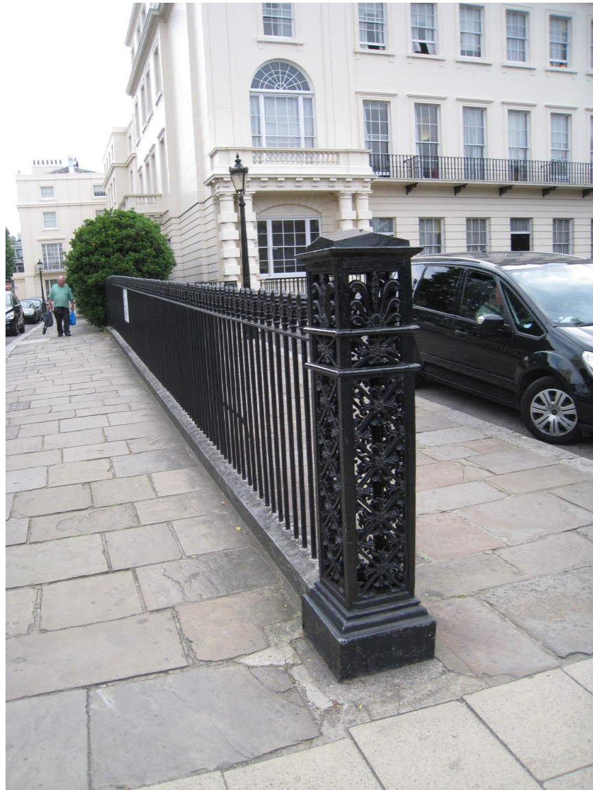
Photo no. 12 Box standard Listed Railings RL14 (part of EH list entry no. 1244298)
