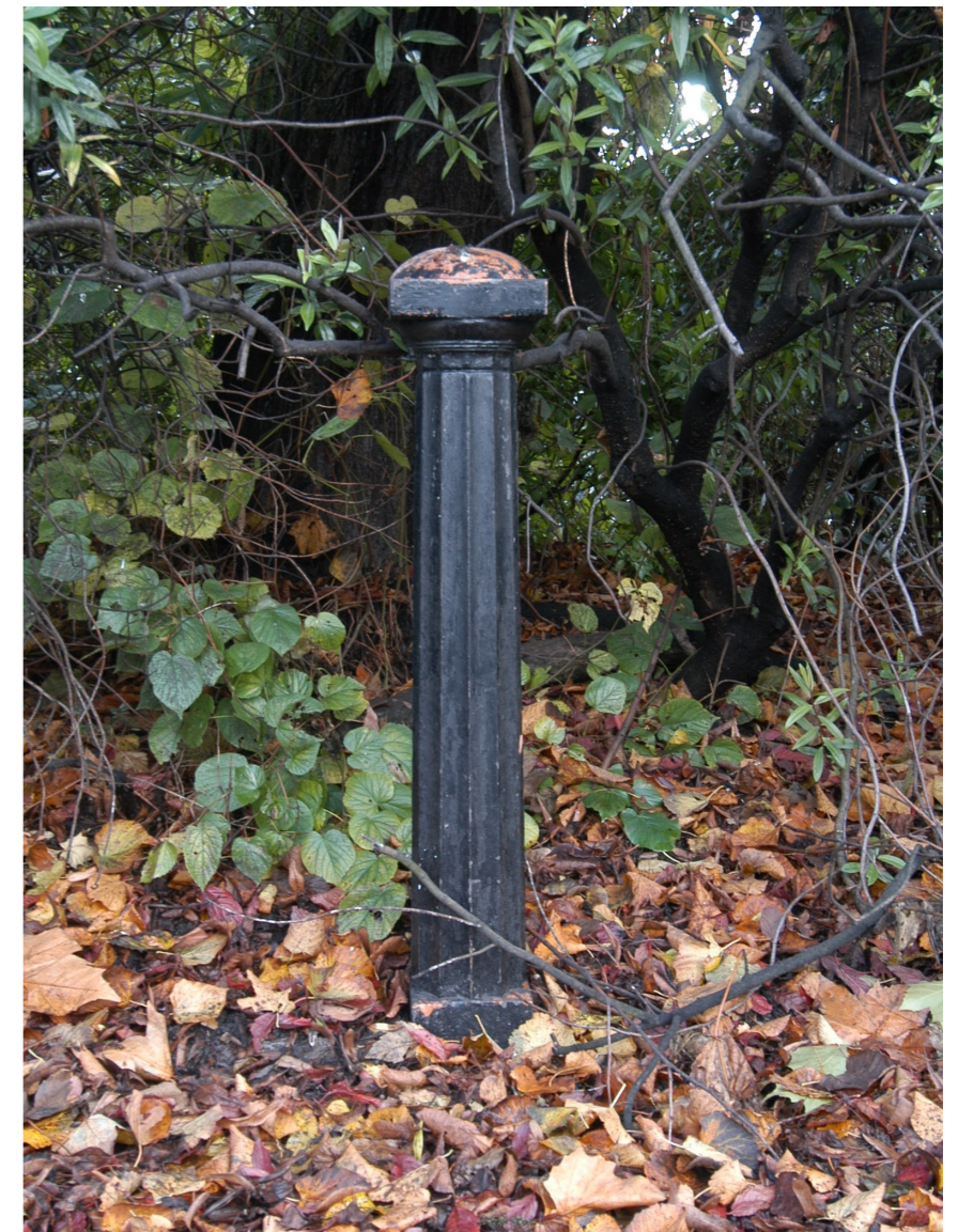
Photo no. 3 Listed bollard BL03 (part of EH list entry no. 1244299)
