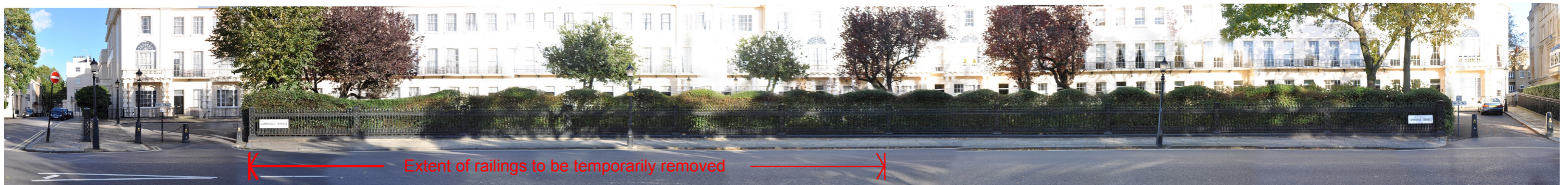
Photo no. 7 Listed Railings RL15 (part of EH list entry no. 1244298)
