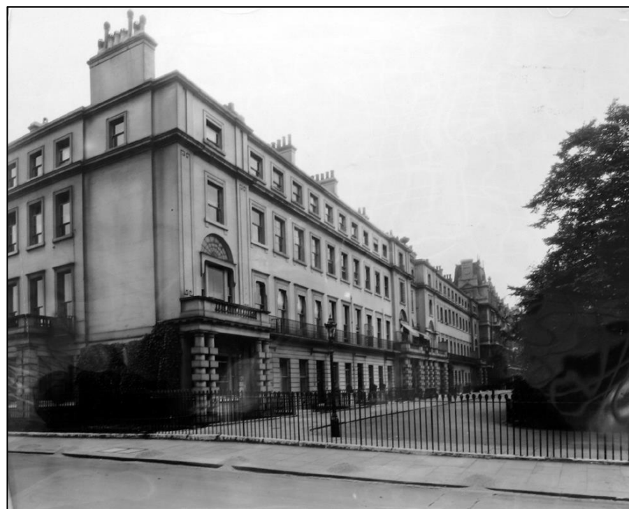
Figure 3.6: View looking south from Chester Gate toward Cambridge Terrace in 1937.
