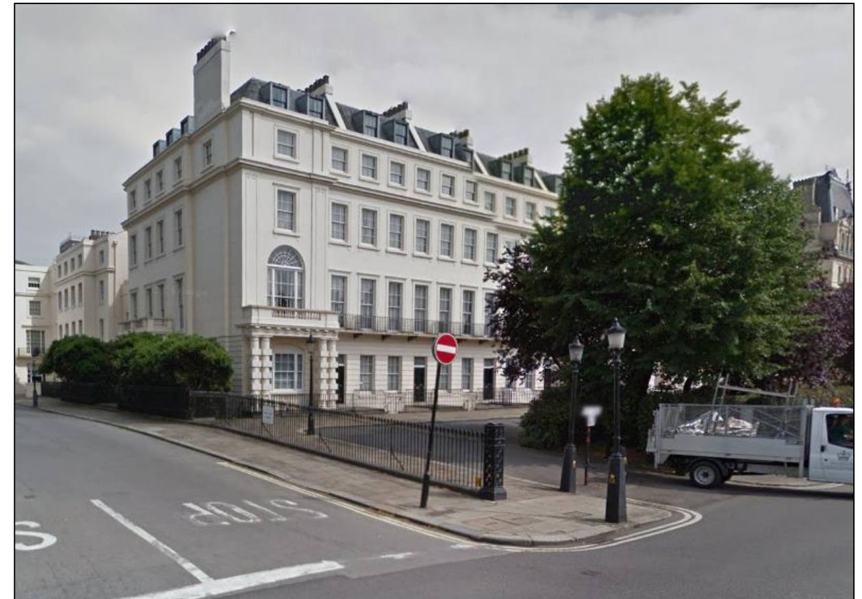
Figure 1.2 View from the Outer Circle looking east towards the Site
