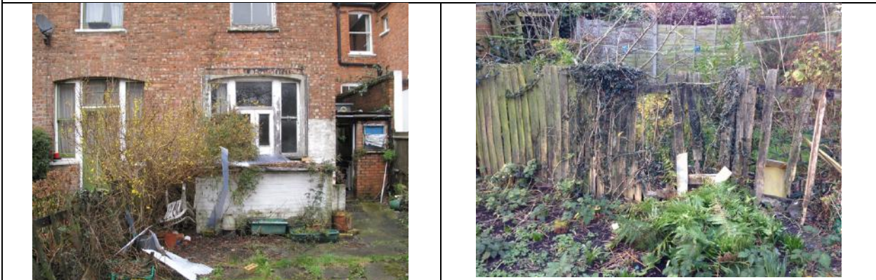
View of the ground floor façade and of the partially collapsed wooden fence separating the property from 15 Chester Road
