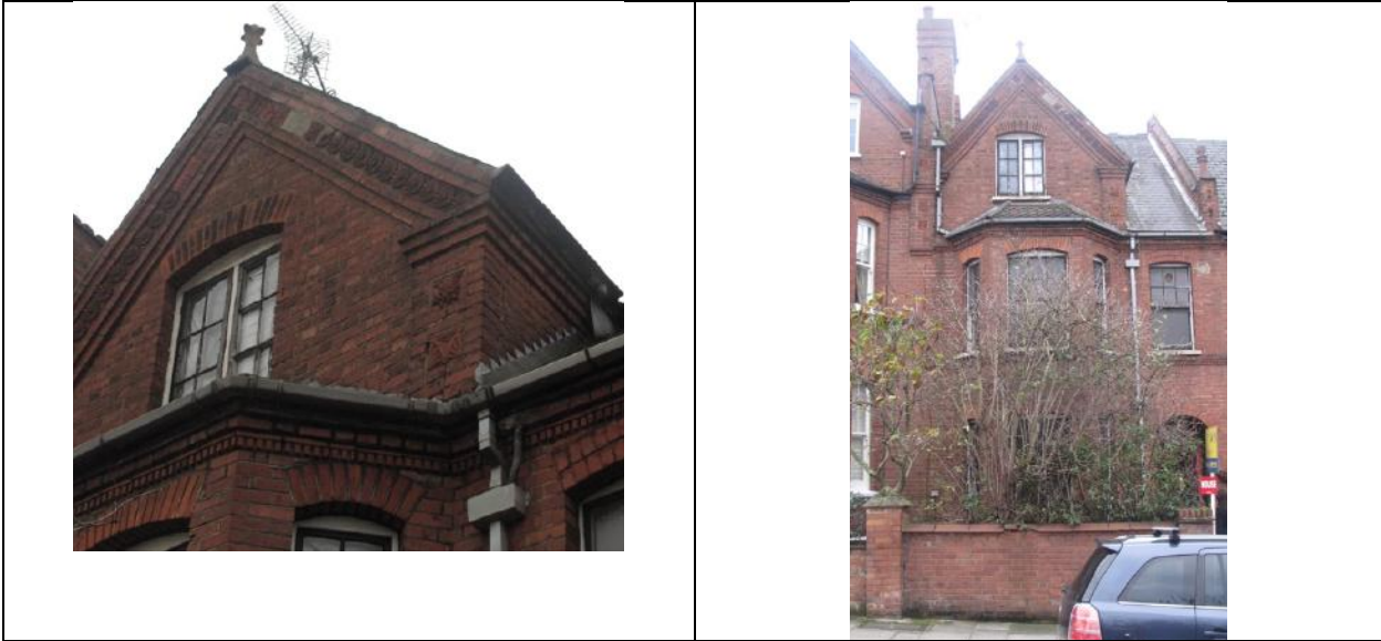
Views of the front façade from Chester Road
