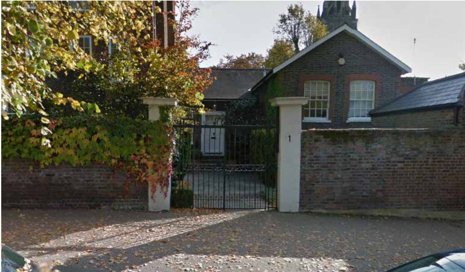
No. 1 entrance gate showing failing pier to the right hand side.
