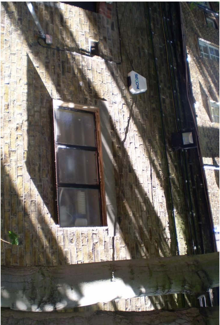
Plate 15 – Repaint to rear elevation of main wall to adjacent property
