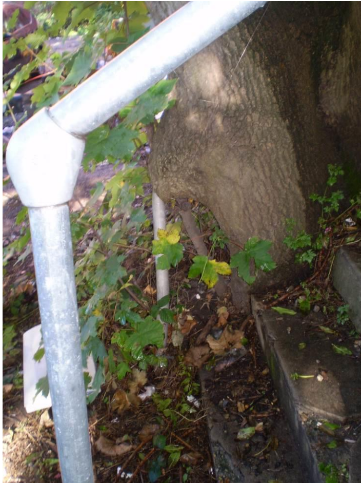
Plate 9 – View of existing hand rail encased by the tree at the steps to 171A
