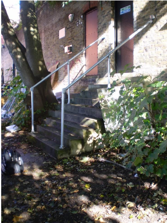
Plate 5 – View of rear access steps to adjoining property
