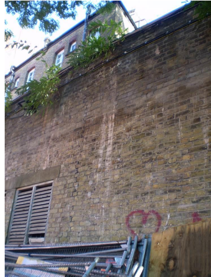
Plate 10 – Vertical crack damage to the rear wall of N° 171A Basement
