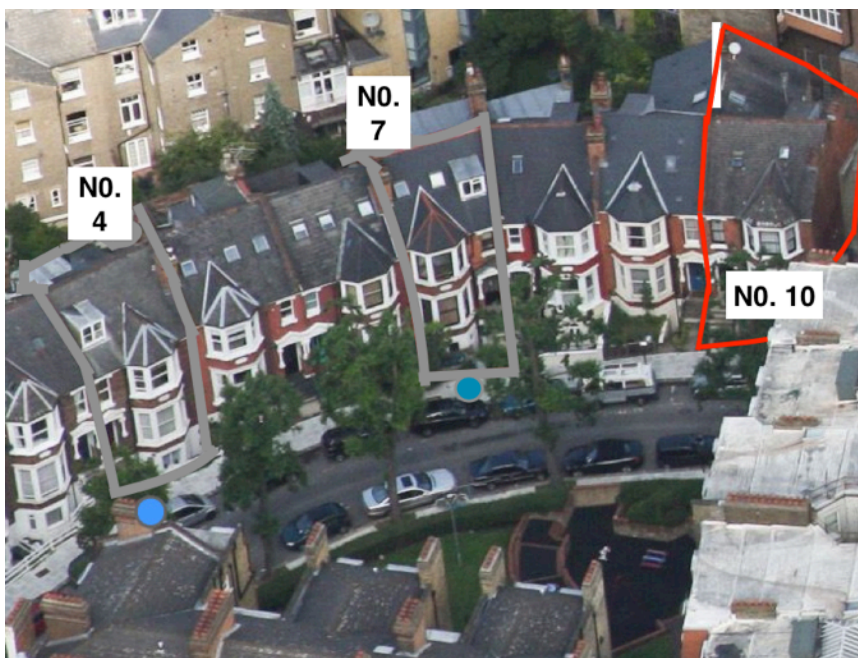
Fig 5 - View of front dormers on Sandwell Crescent
