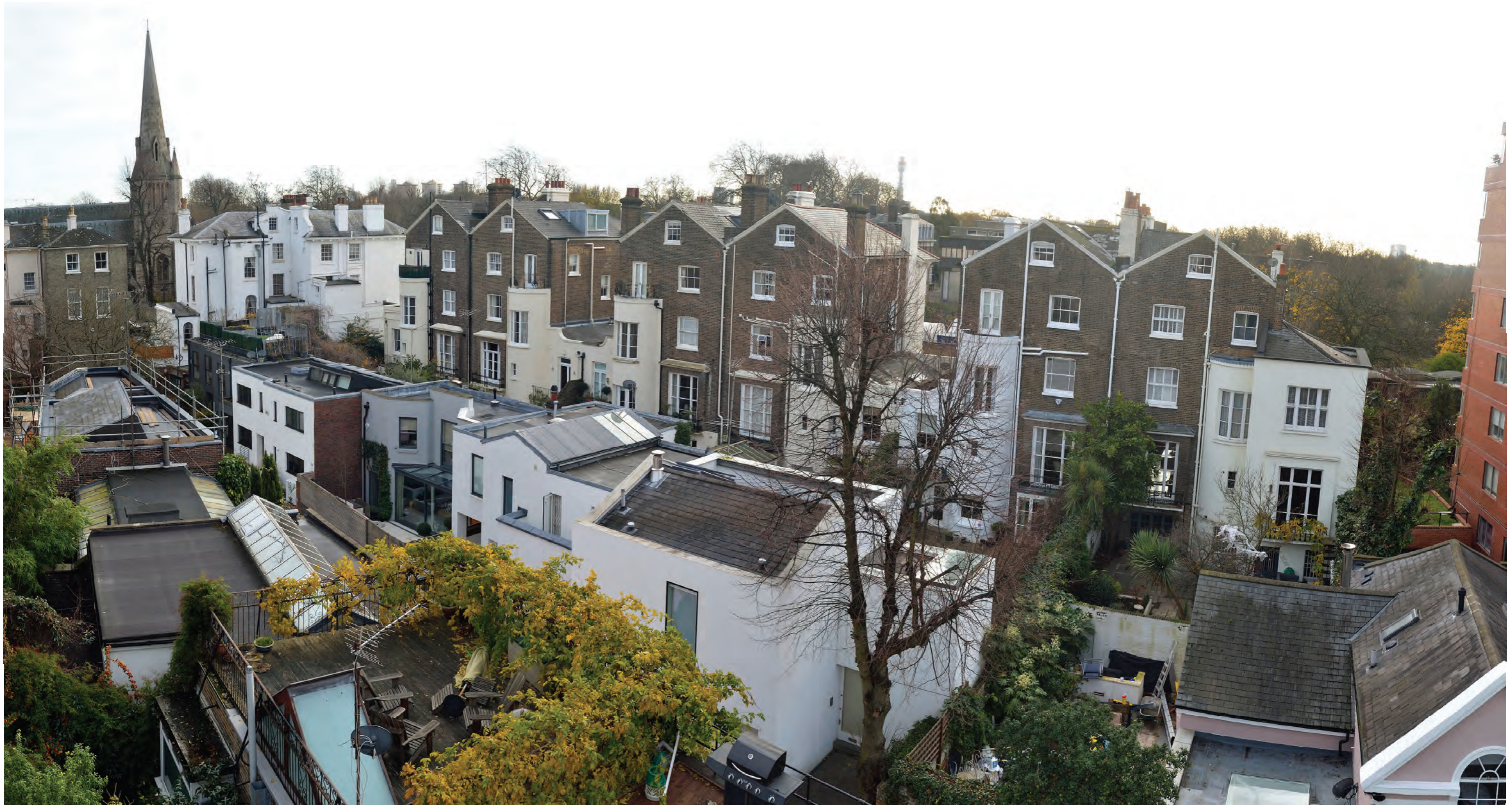
Figure 3.10 A View of 20 Albert Terrace Mews from North West as existing
