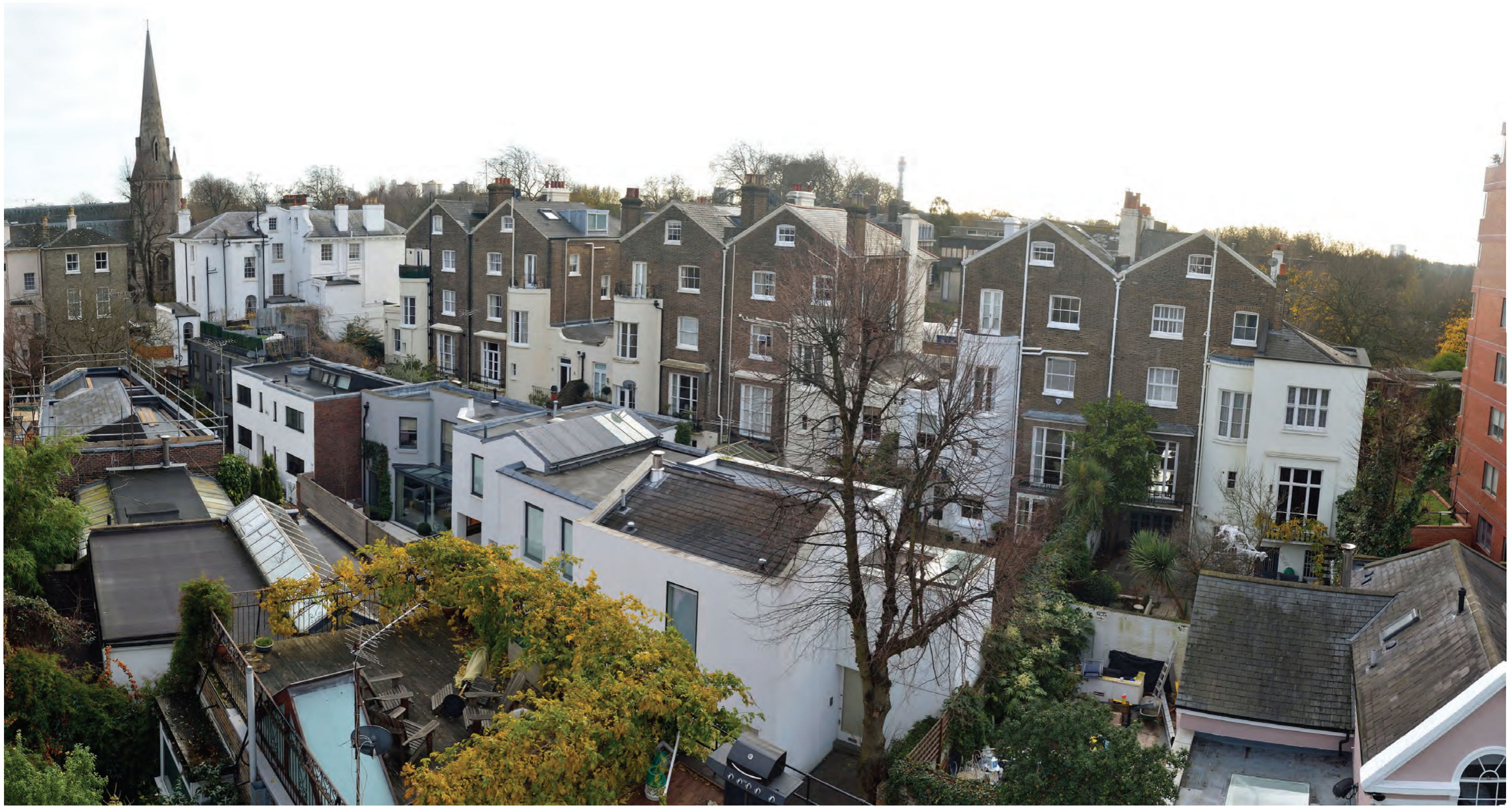
Figure 3.10 B View of 20 Albert Terrace Mews from North West as per permitted scheme 2015/0485/P
