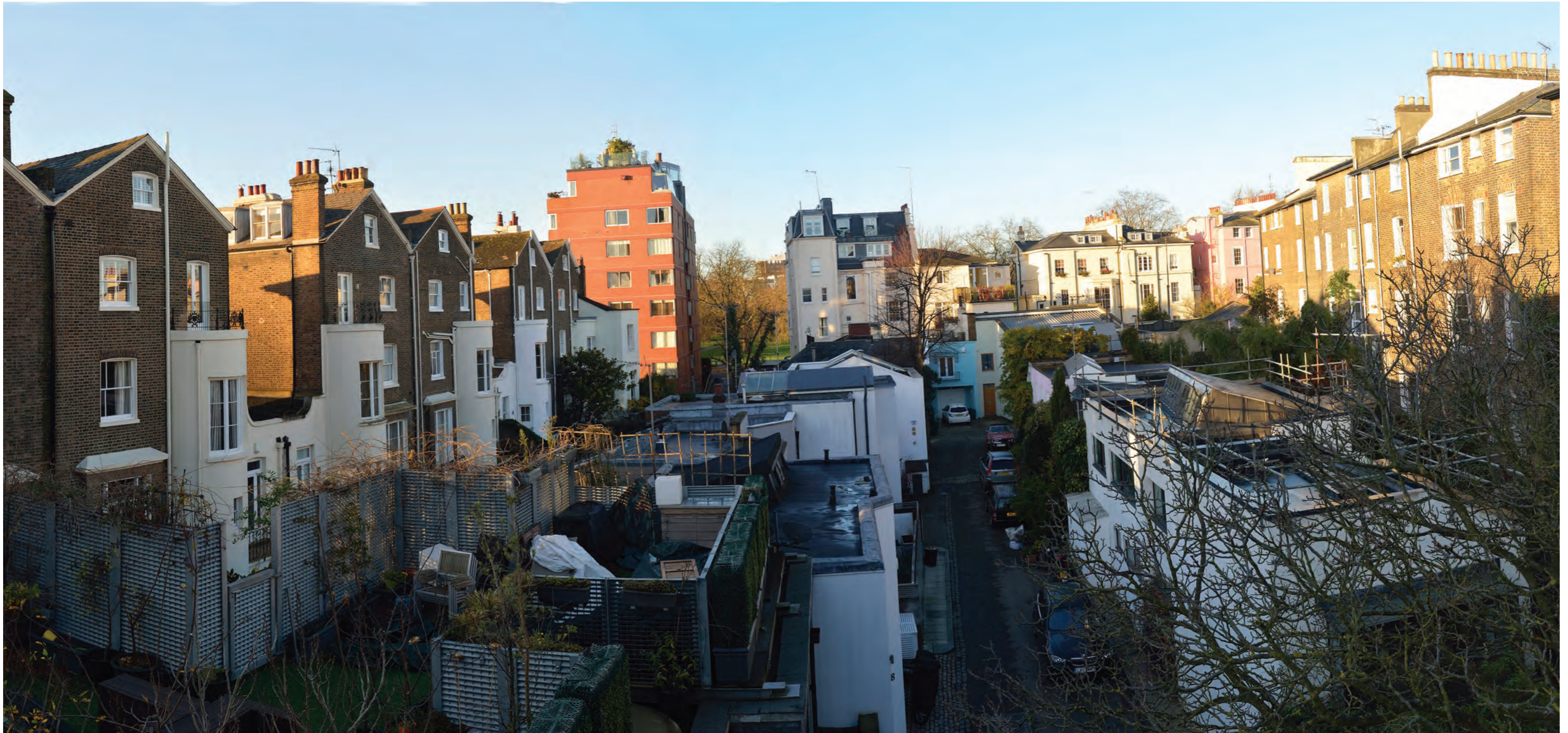
Figure 3.12 B View of 20 Albert Terrace Mews from East as permitted scheme 2015/0485/P
