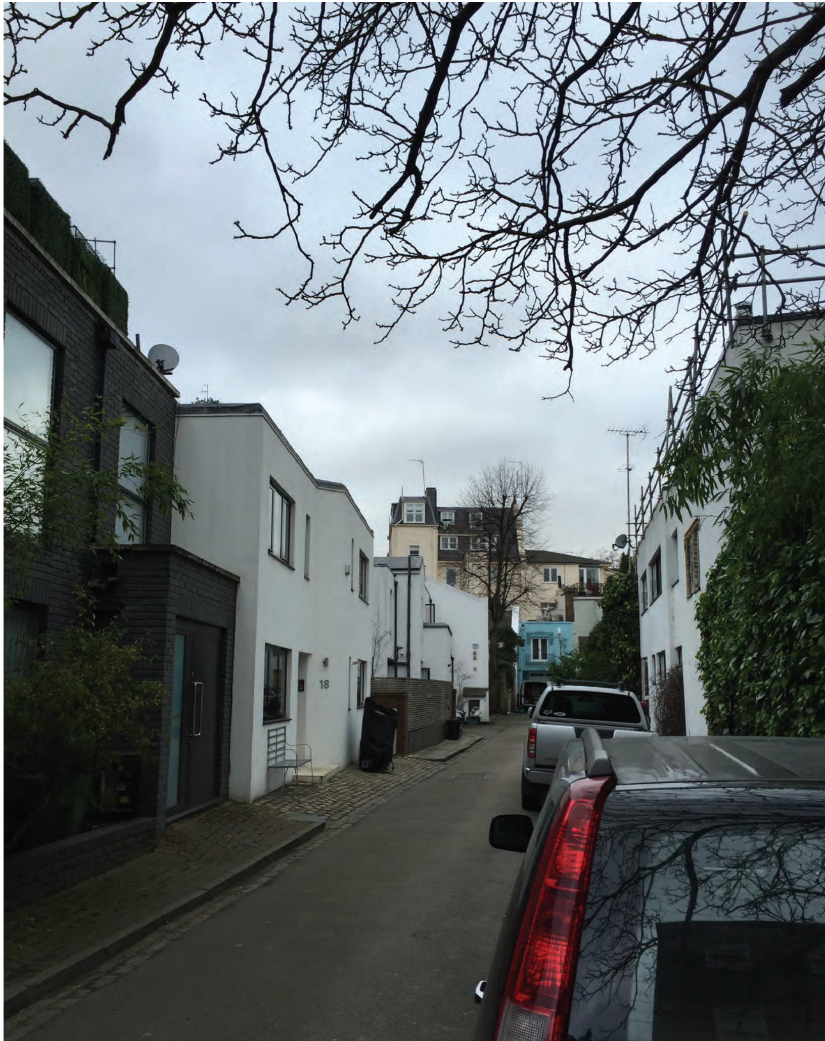
Figure 3.8 A Street view of 20 Albert Terrace Mews from the East as existing
