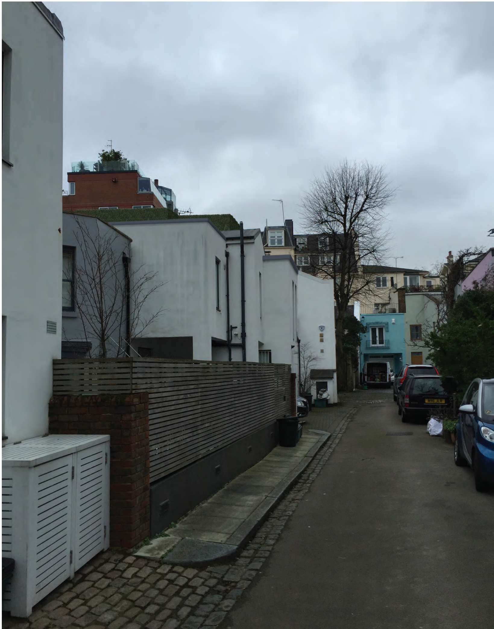
Figure 3.9 C Street view of 20 Albert Terrace Mews from the East as proposed
