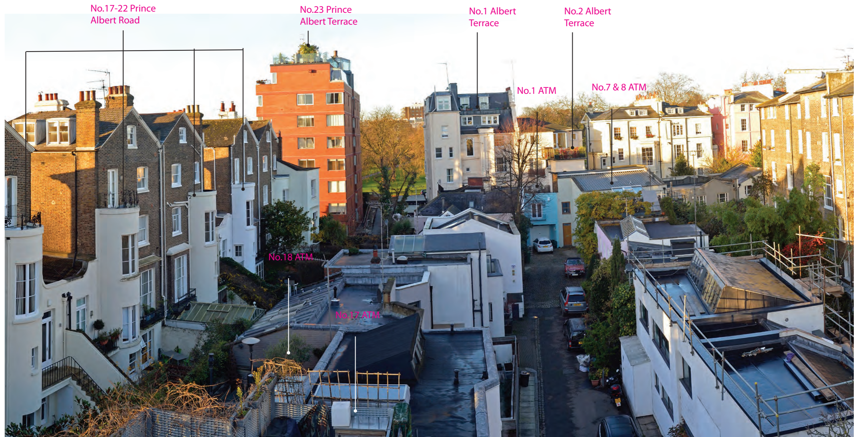
Figure 3.4 J Aerial view of the mews from East
