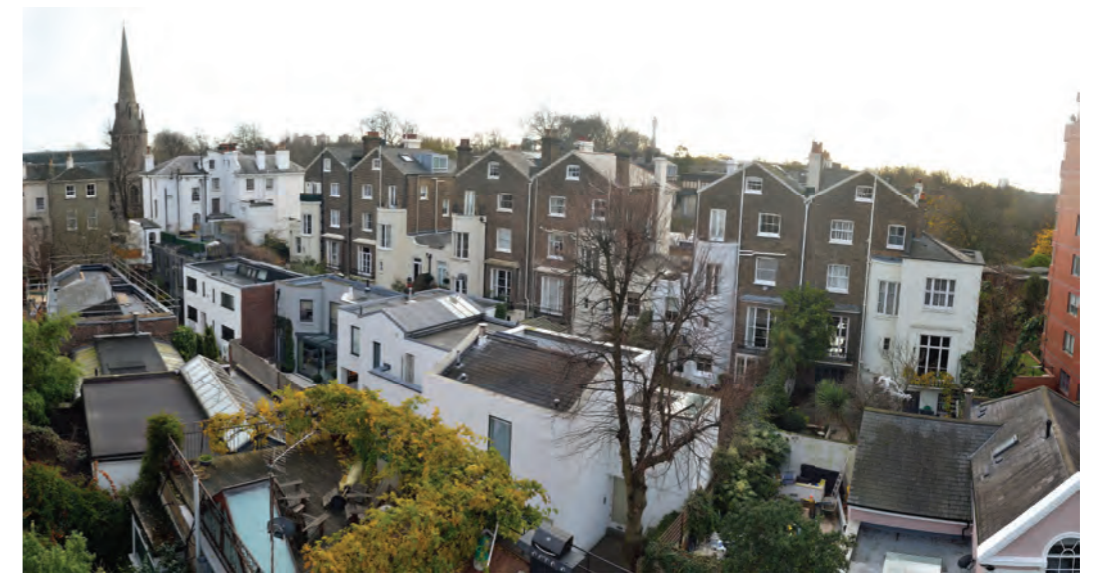
Figure 2.2 Aerial image of the mews from North West
