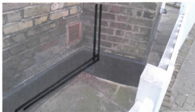
Figure 2: Downpipe and horizontal pipe
