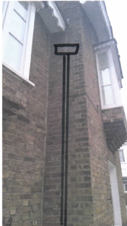
Figure 1: Downpipe and hopper
