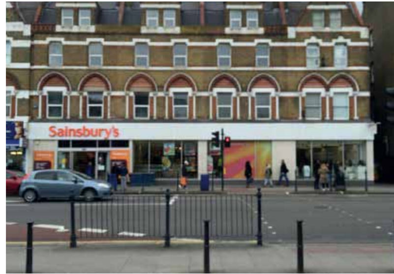
Photo of existing
