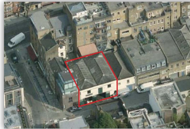
Figure 4 20-21 King's Mews Aerial View
