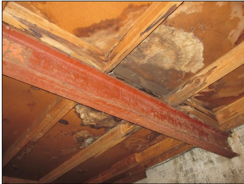
5. Extensive damp staining and suspected wet rot to first floor ceiling structure.
