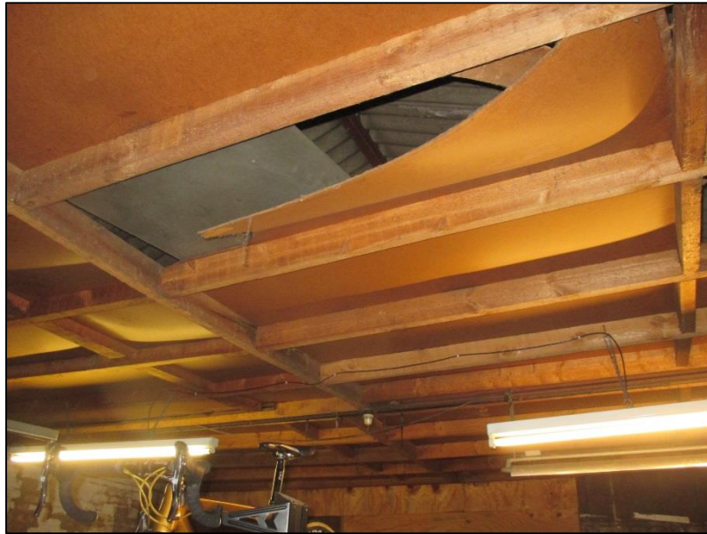
7. Displaced ceiling finish to first floor.
