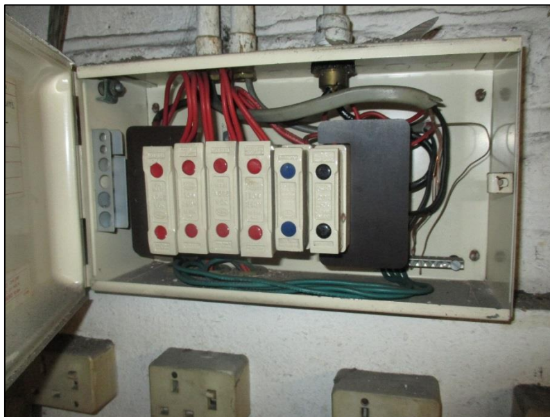
17. Dated electrical fusebox to RH wall at first floor level.
