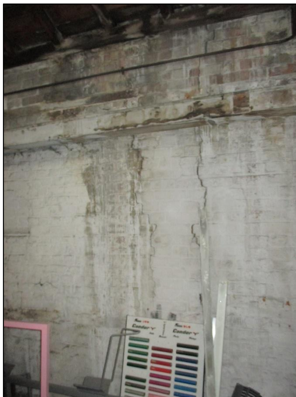
14. Vertical cracks to LH party wall at first floor level.
