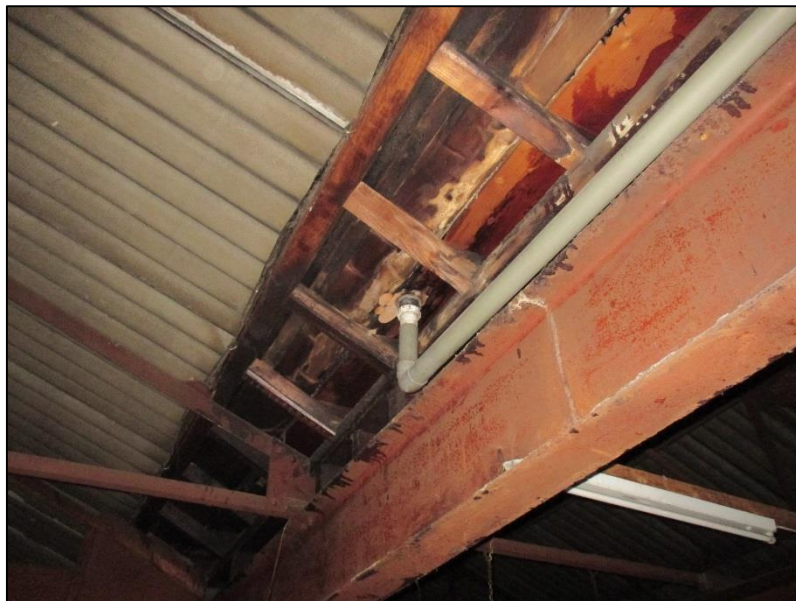
8. Damp staining to underside of central valley gutter with waste pipe connection.
