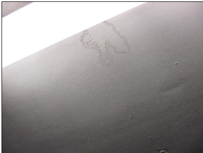
6. Fibrous cement boarding to ground floor ceiling finish.
