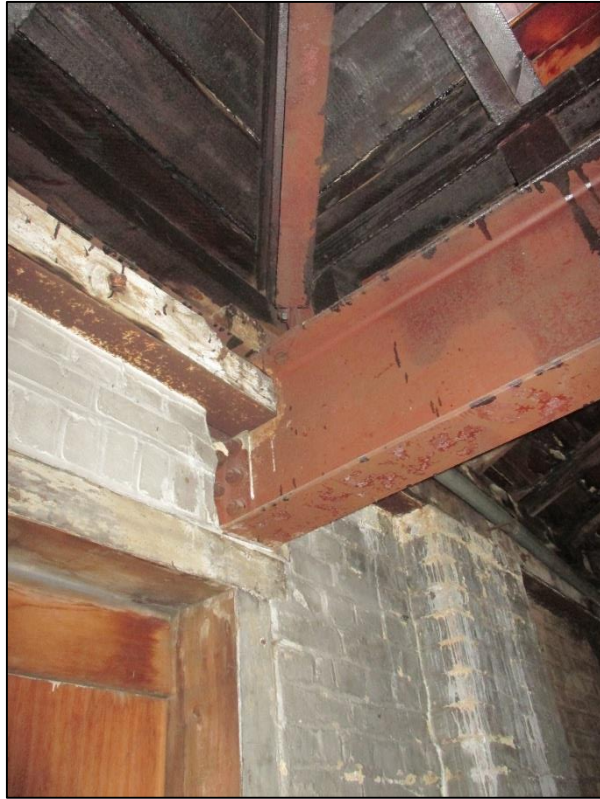
11. Steel beam supported upon timber door frame/lintel.
