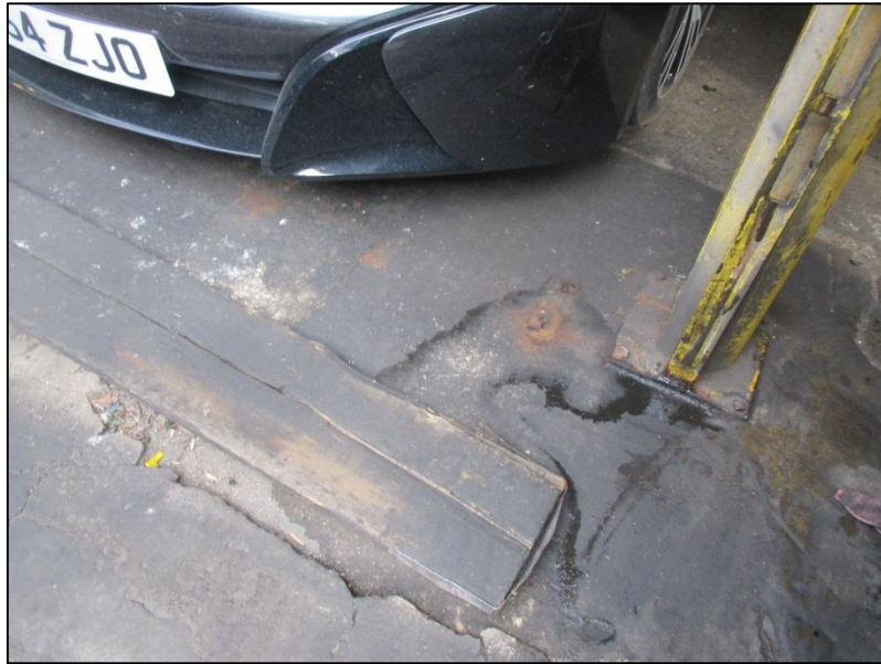
15. Damaged ground floor slab at door threshold location.
