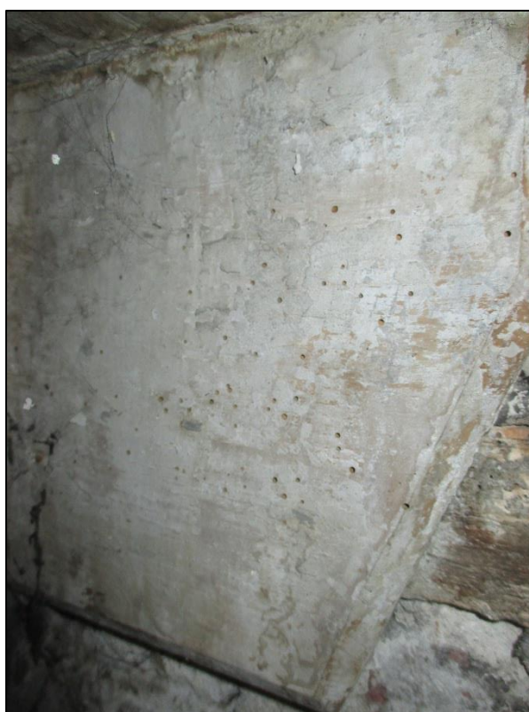
22. Woodboring insect attack to rear wall.
