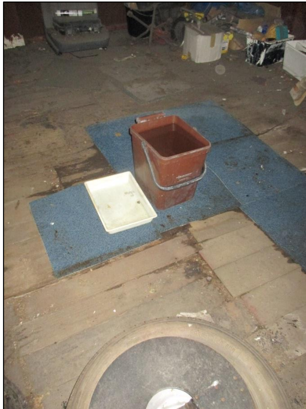
9. Accumulated water below central valley gutter.
