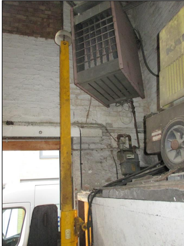
19. Gas heater and gas meter to workshop.
