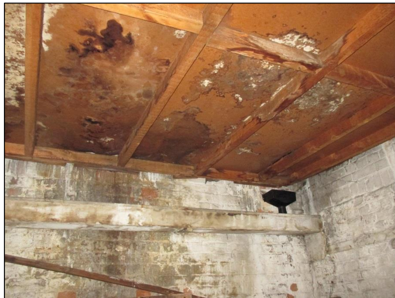
10. Further decay to first floor ceiling surface.
