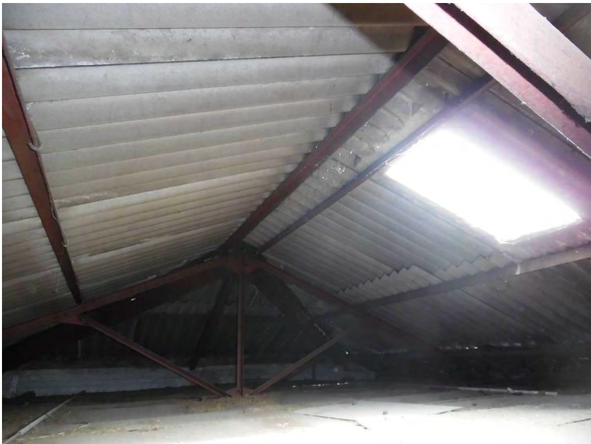
Fig.19 Detail of roof interior (1)
