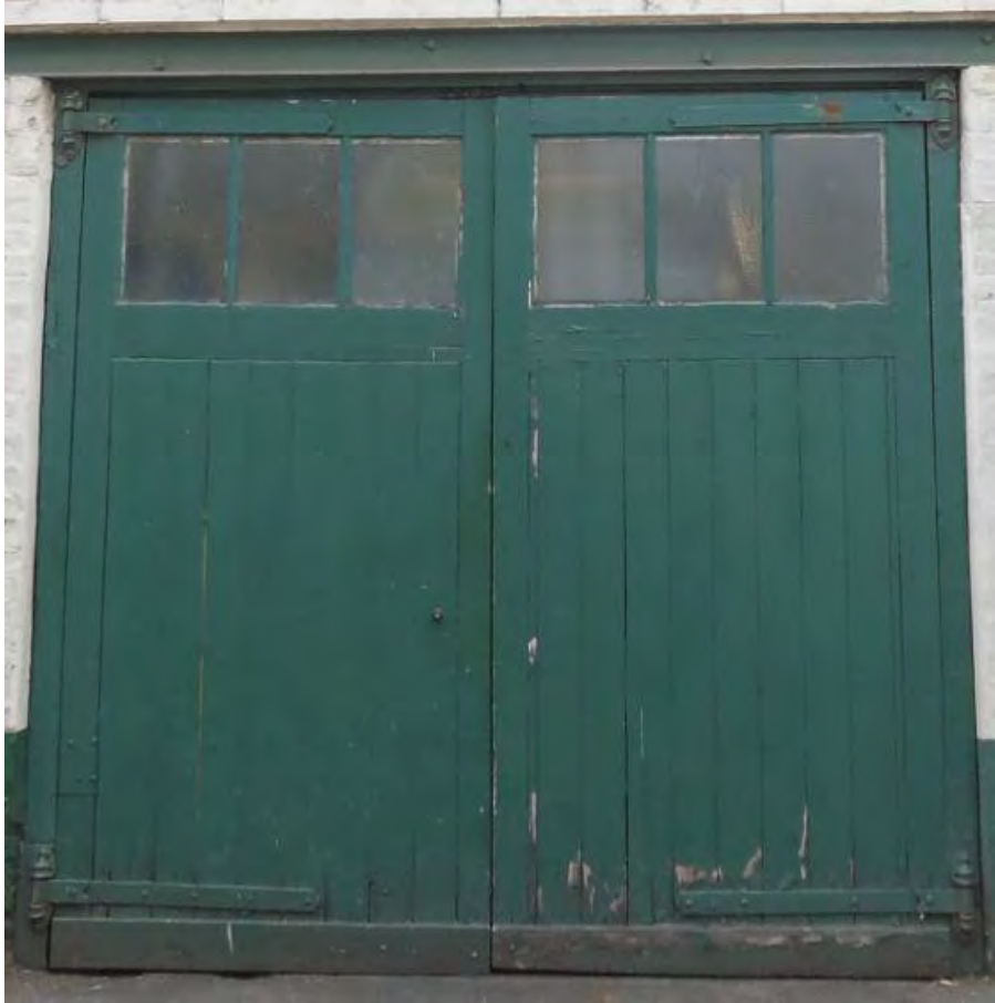
Fig.16 Detail of Collinge's hinges
