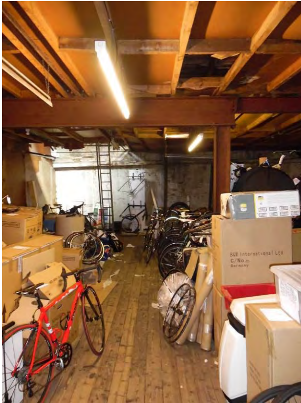
Fig.35 First floor rear open plan space looking north
