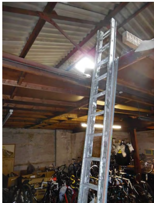
Fig.36 First floor rear open plan space, platform to roof void
