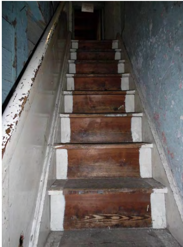
Fig.26 Straight flight timber staircase leading to the first floor
