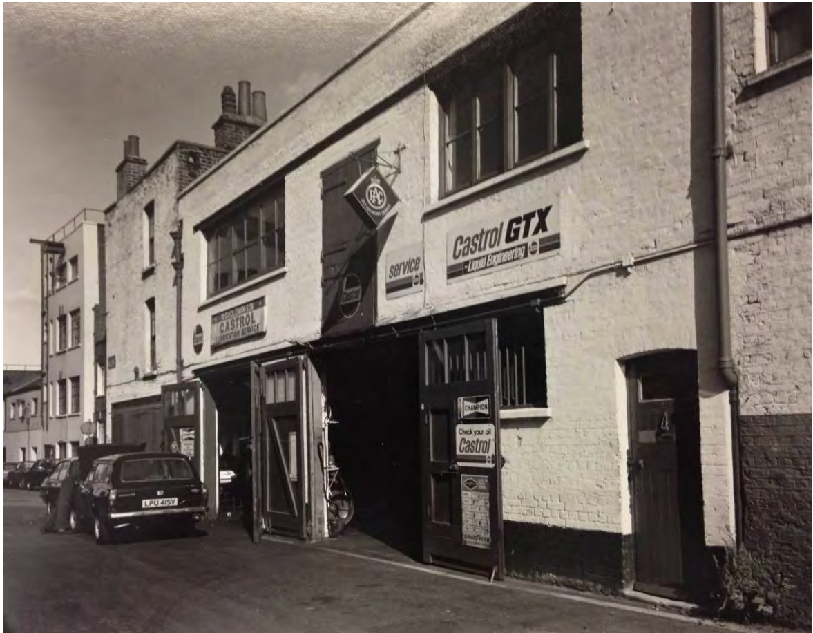
Fig.15 A photograph of the building in 1980 (Camden Archives, ref: 89.3 KM, 032325, Neg.755. P.D. Barkshire)
