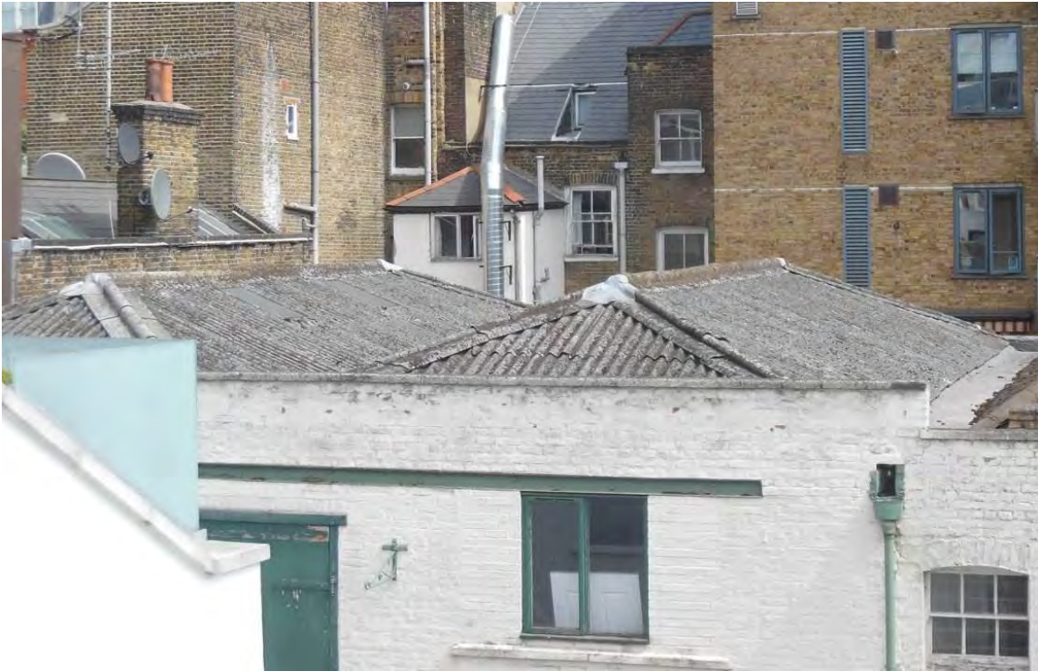
Fig.18 Detail of roof
