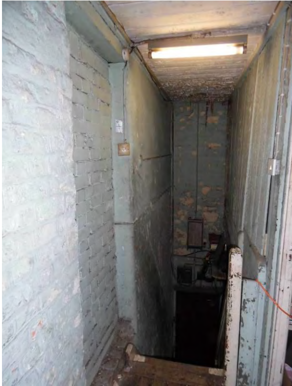
Fig.27 First floor landing looking down the staircase
