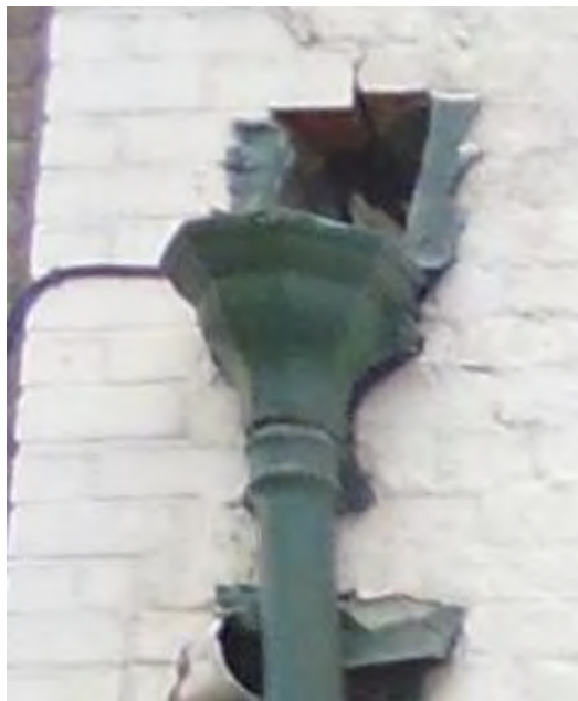
Fig.17 Detail of cast-iron hopper head
