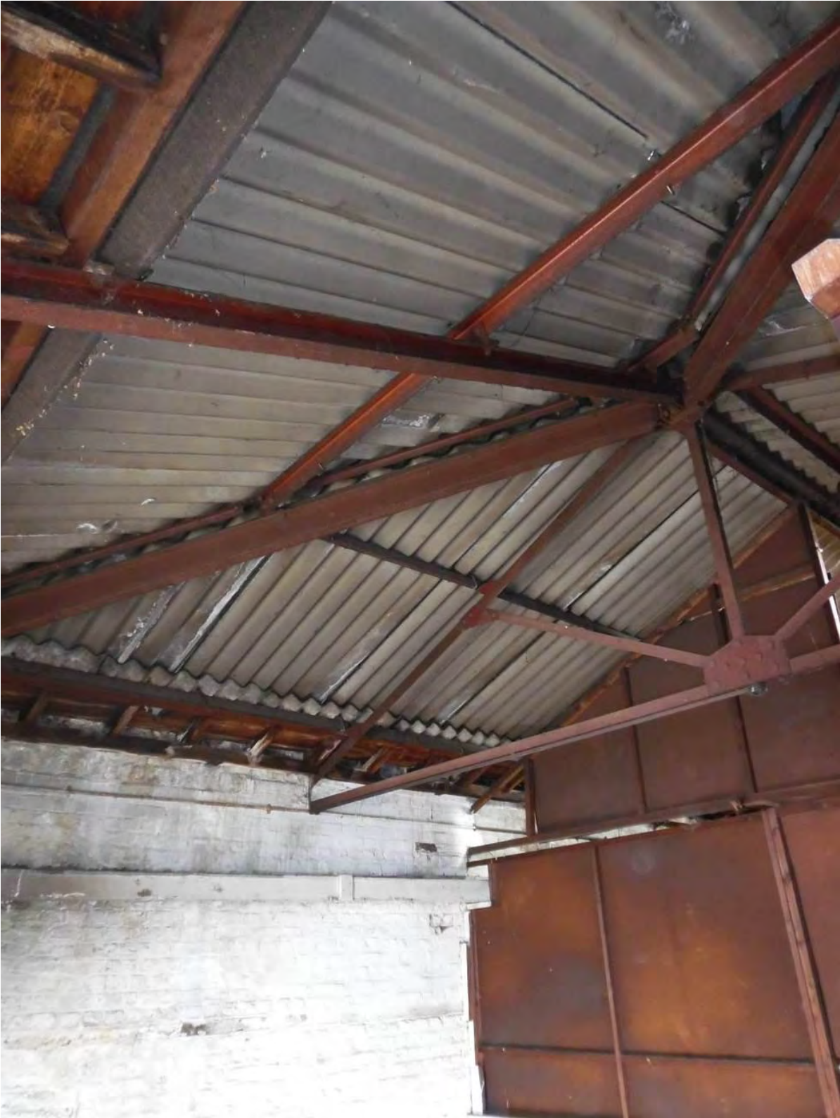
Fig.20 Detail of roof interior (2)
