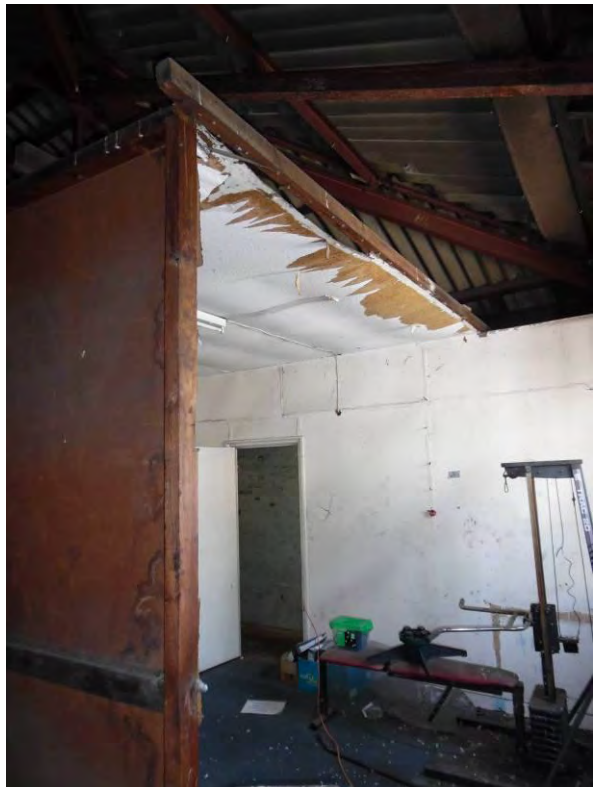
Fig.30 First floor partitioned space at the front of the building looking north-west
