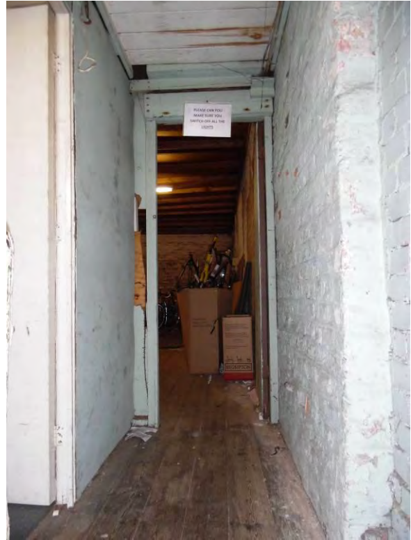
Fig.28 First floor landing looking east
