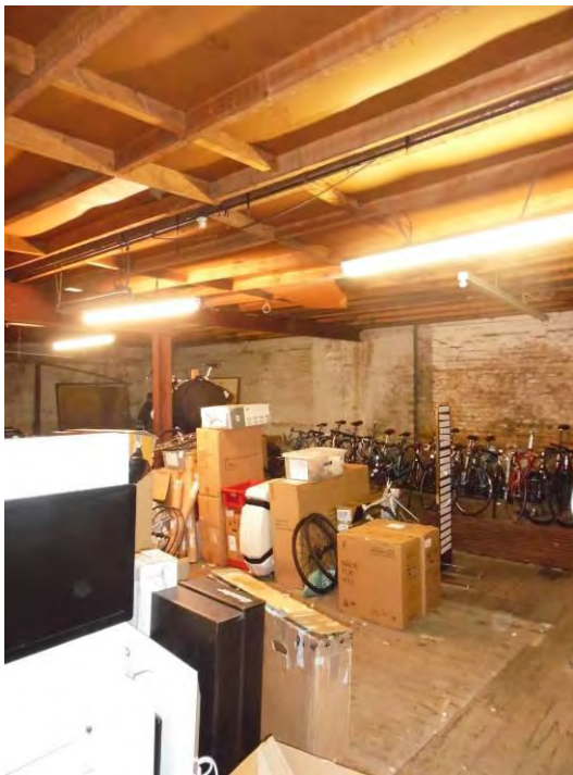
Fig.33 First floor rear open plan space looking north east
