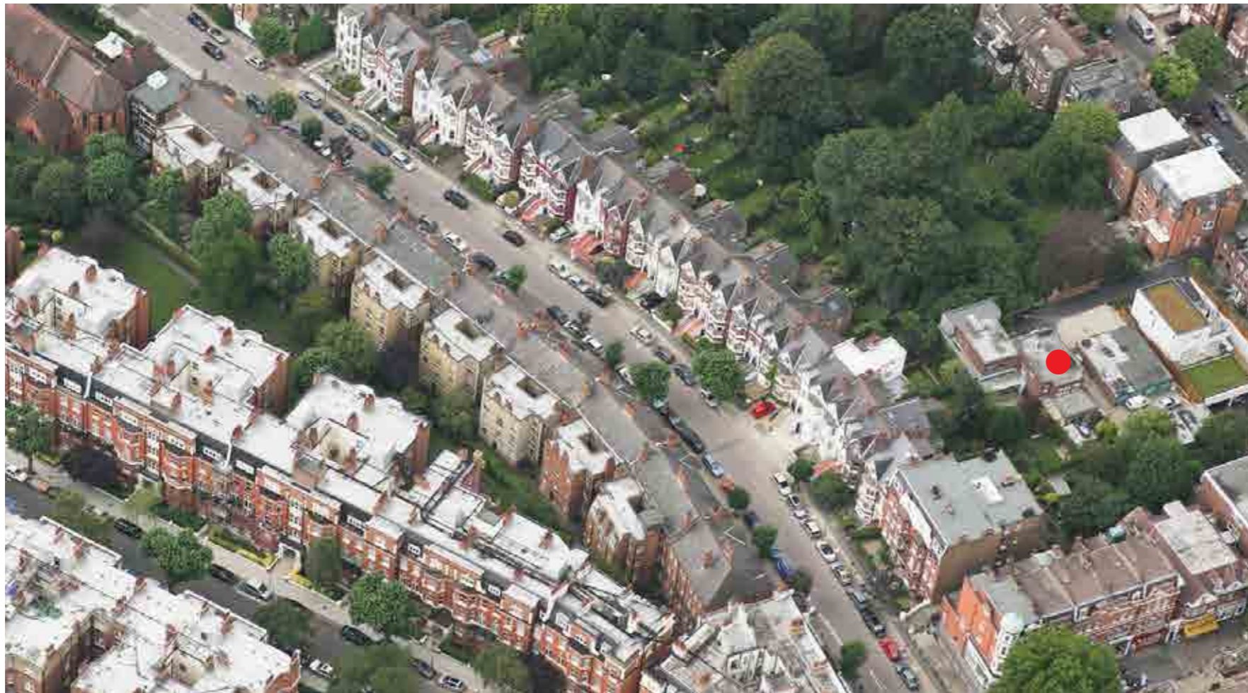
Fig 6 Aerial view of the rear of 1E Parsifal Road (shown by red dot)
