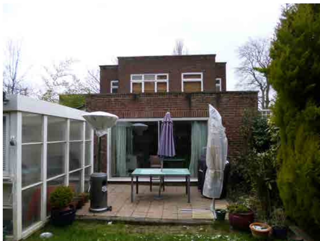
Fig 3 Northeast elevation of 1E Parsifal Road
