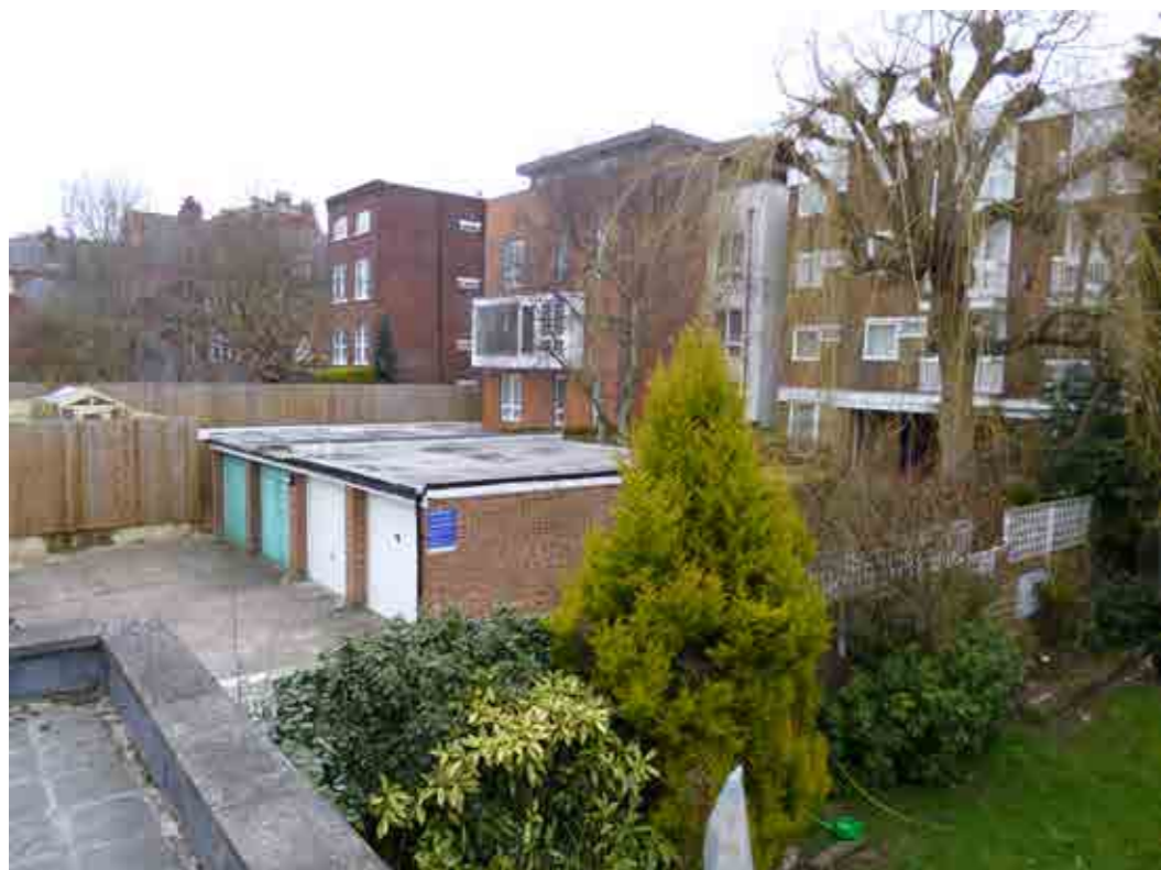
Fig 8 View through neighbour on the northeast
