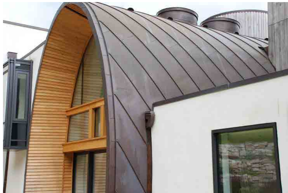
Fig 17 Zinc Cladded Roof
