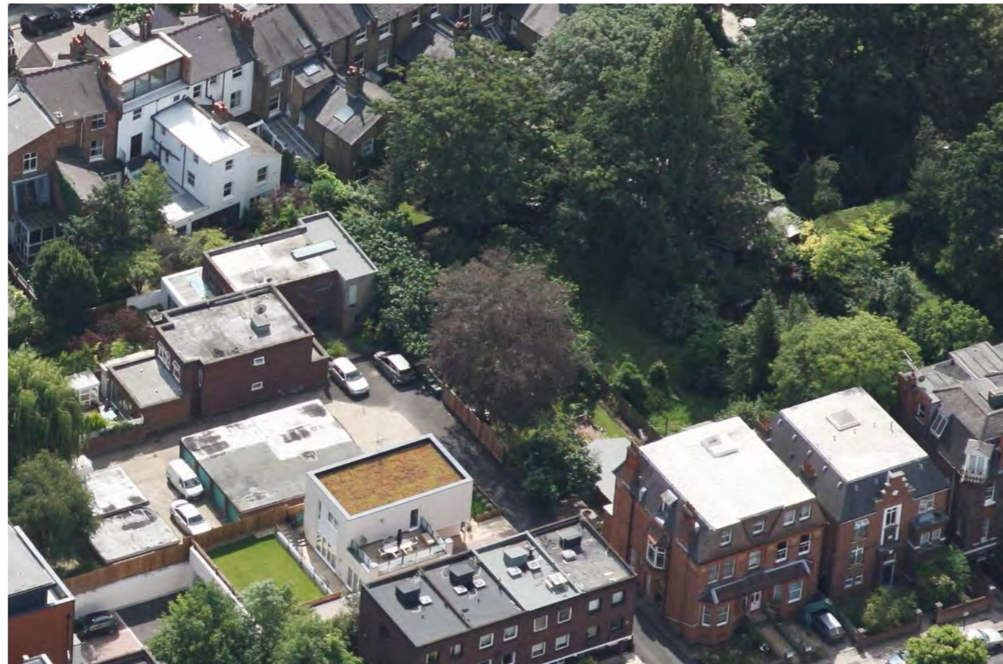
Fig 15 Mansard roof on Parsifal Road
