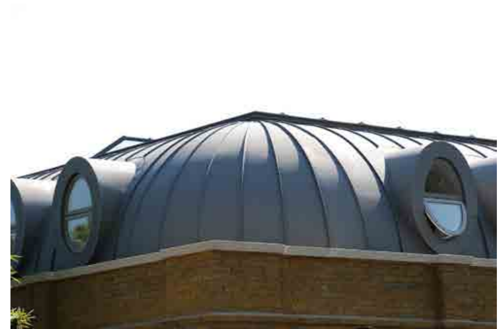
Fig 19 Zinc Mansard Roof
