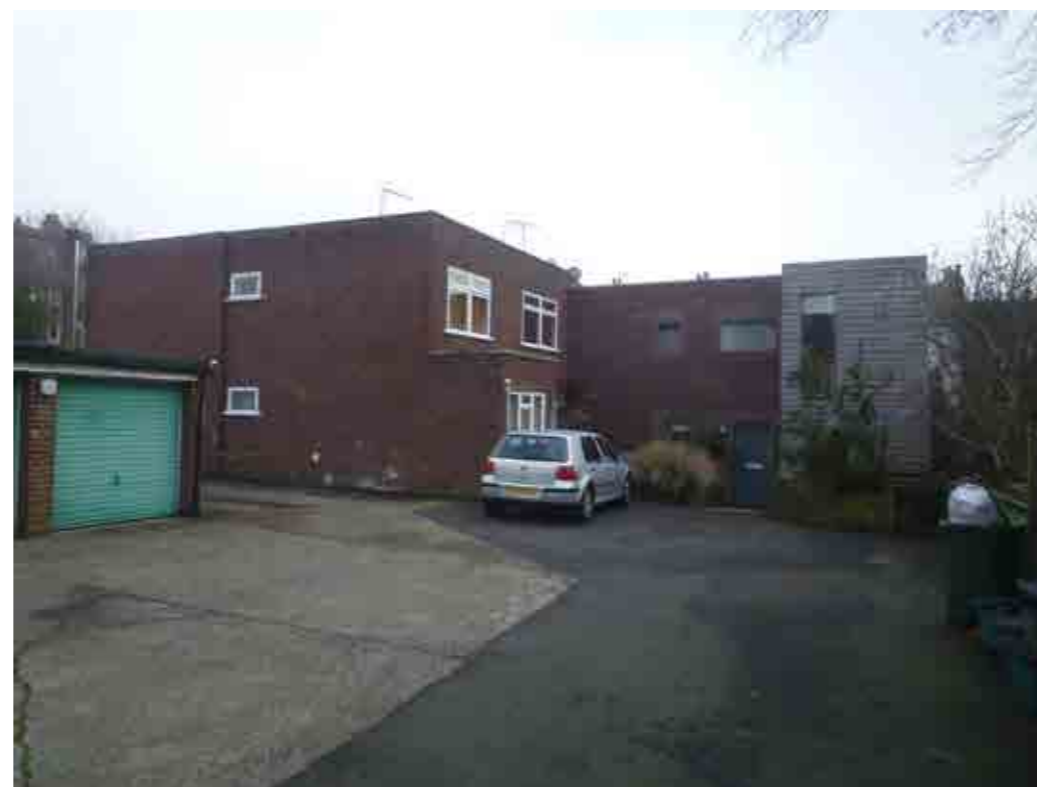
Fig 2 Northwest elevation of No. 1E and 1F Parsifal Road
