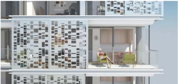
External sliding façade shutters
