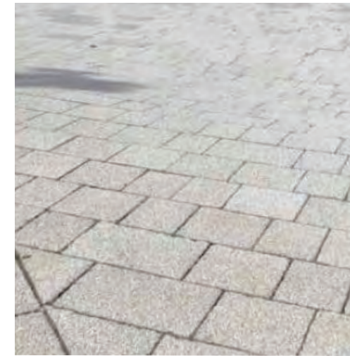
Permeable concrete paving within tree RPA
