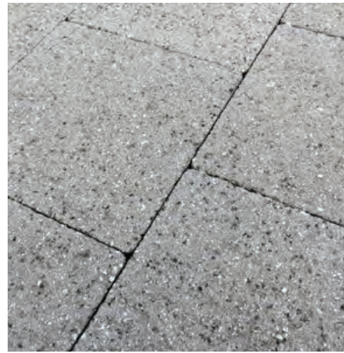
Concrete paving to route to cycle storage
