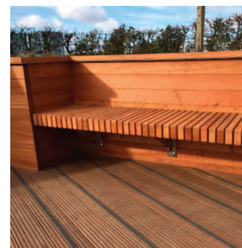
Raised timber planters to amenity area
