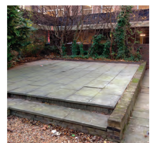
View looking to north-west boundary wall
