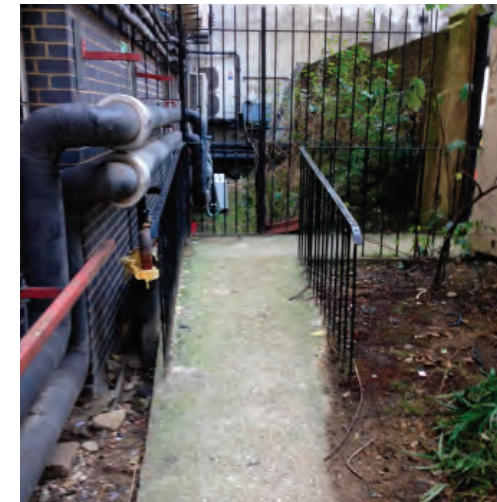
Existing ramp access to Campbell House amenity area
