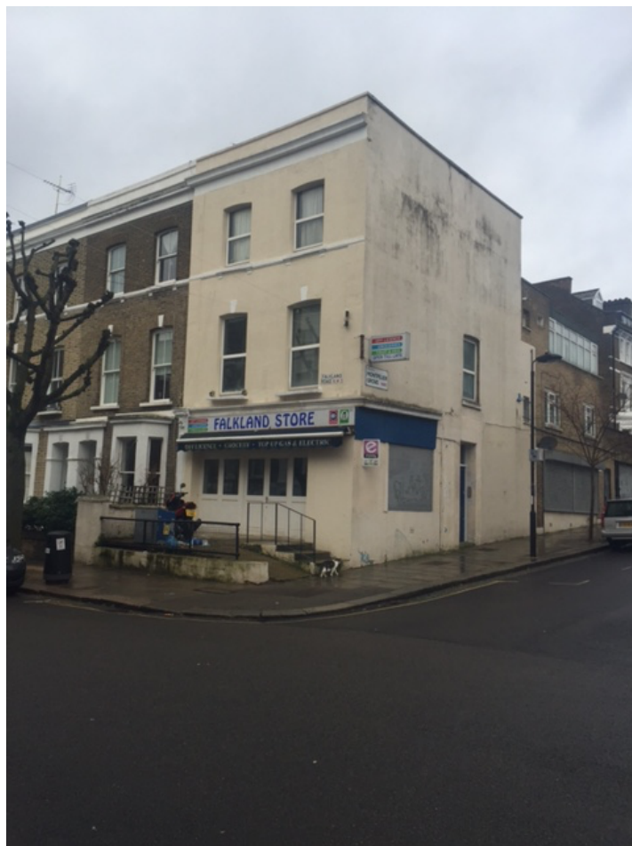
Front and side view from Falkland Road and Montpelier Grove
