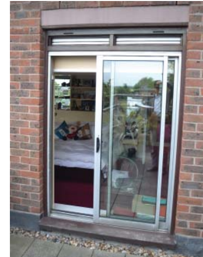
Example of 5th floor aluminium frame double glazed door, size and style to match existing
