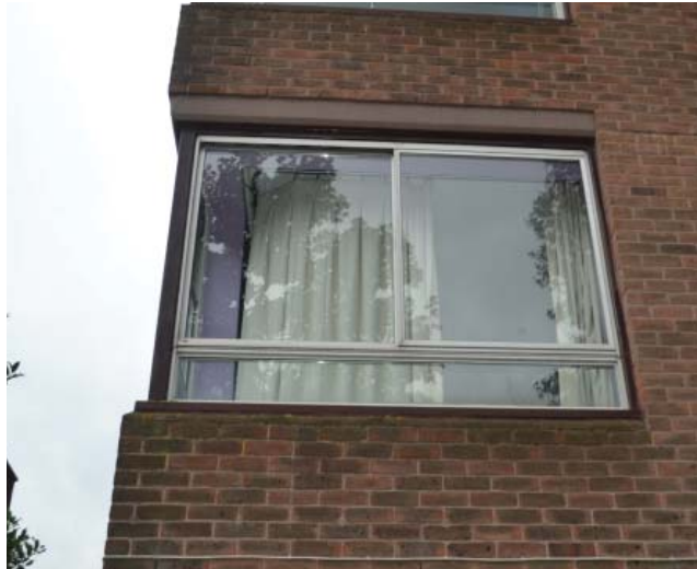
Example of 5th floor aluminium frame double glazed windows and existing brickwork to match existing
