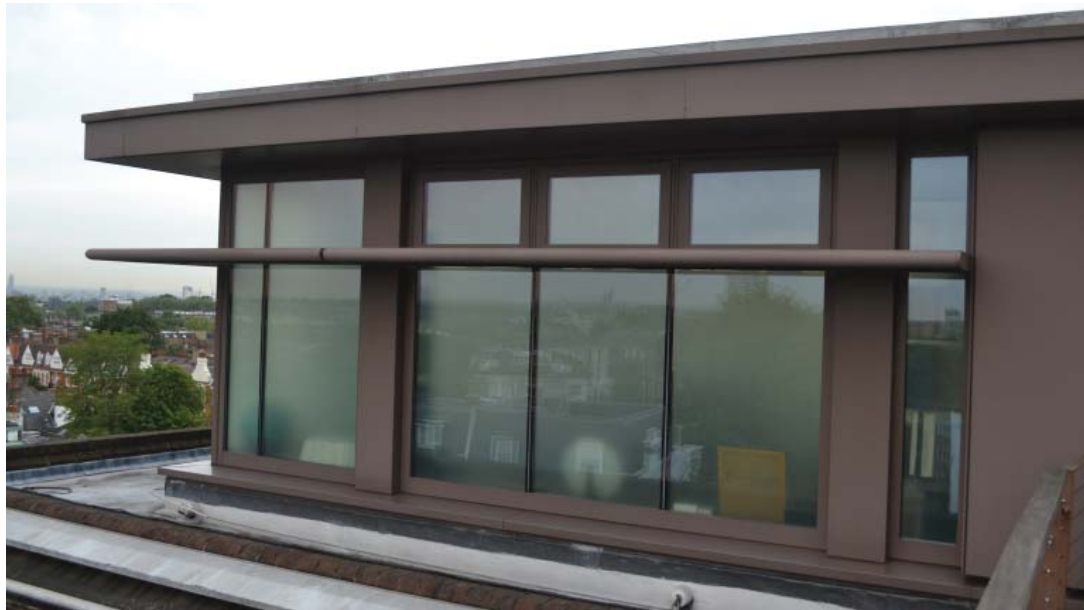
Example of 6th floor double glazed windows and powder coated metal frame colour brown BS 4800 (08B25). The colour of the proposed 6th floor extension will match existing.
