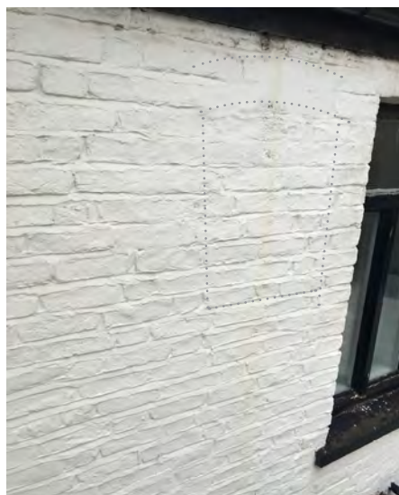
Fig 14. Detail from closet wing extension Evidence of a brick arch from an infilled window from a previous time
