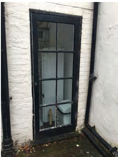
Fig 13. Detail from closet wing extension elevation to the rear: note concrete lintel over the door indicating that it is a new addition
