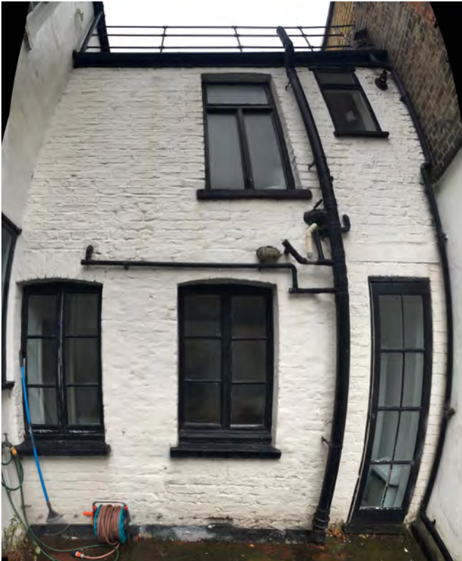
Fig 11. Closet wing extension elevation to the rear - Note concrete lintel over the doorway, indicating that it was not inserted in Victorian times.
