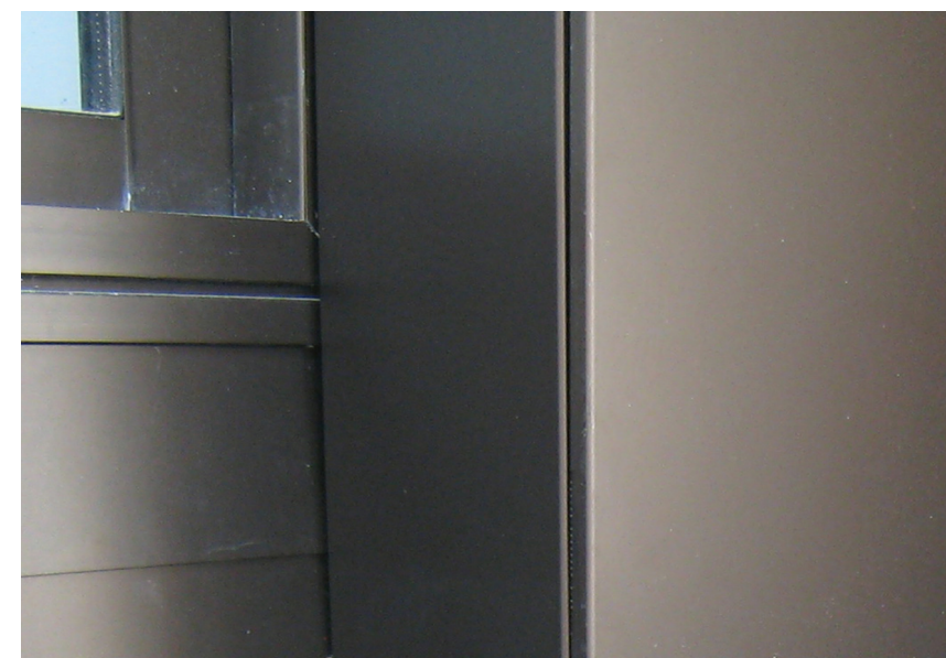
2 - Aluminium with Bronze finish to illustrate proposed colour of Aluminium glazing frames
