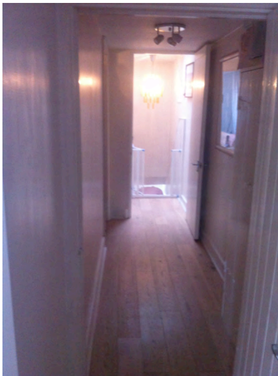
Existing Corridor at First Floor
