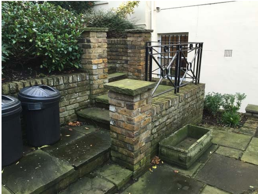
Photograph 2: Level changes and hard landscaping between T5&6 and likely footprint
