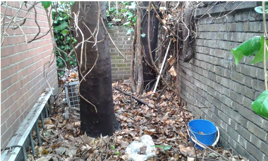
Photoview 2: illustrating proximity of T1 (left of frame) and T2 to laundry room wall (left of frame) and boundary wall
