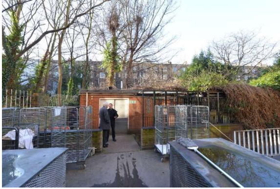
Figure 2 – Existing laundry outbuilding – East Elevation
